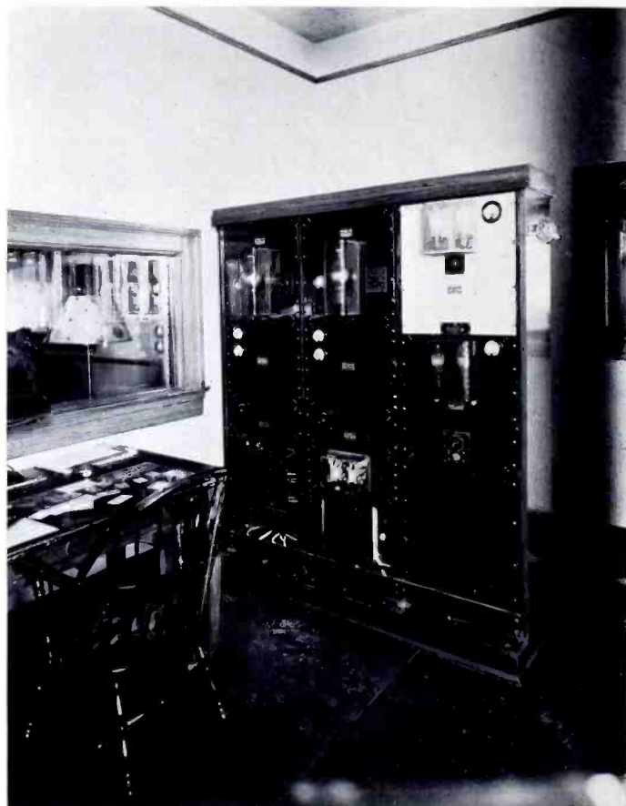
WTAR, NORFOLK, VA.—POWER SUPPLY RECTIFIERS AND FILTERS. STUDIO MASTER CONTROL ROOM, SHOWING TWO 12-VOLT, 10-AMPERE FILAMENT RECTIFIERS AND TWO 350-VOLT PLATE RECTIFIERS, USING 866-A TUBES. NOTE—THE PAIR OF 866 TUBES IN THE TOP OF THE 350-VOLT UNIT LASTED 8,000 HOURS AND WERE STILL GOOD WHEN REMOVED. (WE WERE BEGINNING TO FEEL APPREHENSIVE!)
