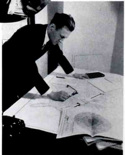
(ABOVE) MEASURING THE COVERAGE AREA OF A RADIO STATION BY THE USE OF A PLANIMETER
