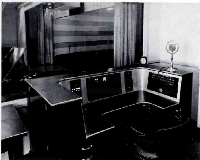
Typical control room which permits full vision into the studio.
