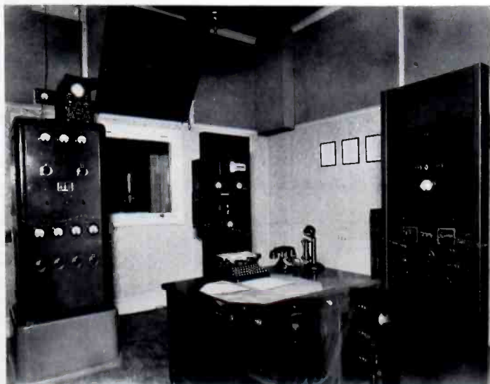
Convenient arrangement of the transmitter and speech input equipment at WRAW.
