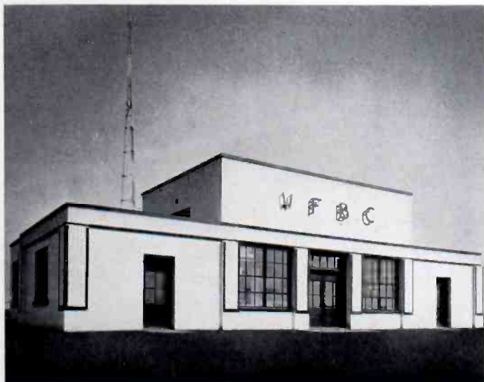
The modern transmitter house.
