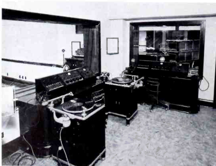
The WKY control room showing the two RCA operator's consoles and turntable equipment.
