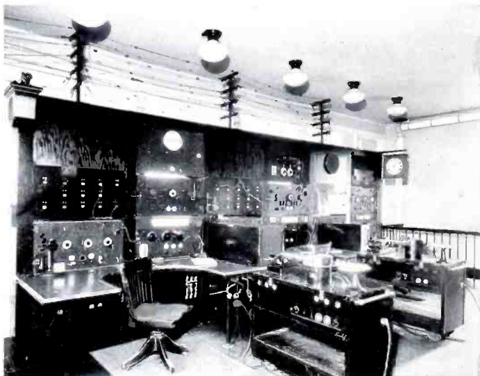
The interior of the RCA Communications Laboratory, Riverhead, Long Island.
