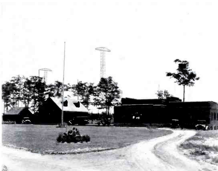
A view of the Research Division and Frequency Measuring Buildings. Marconi towers in the background.
