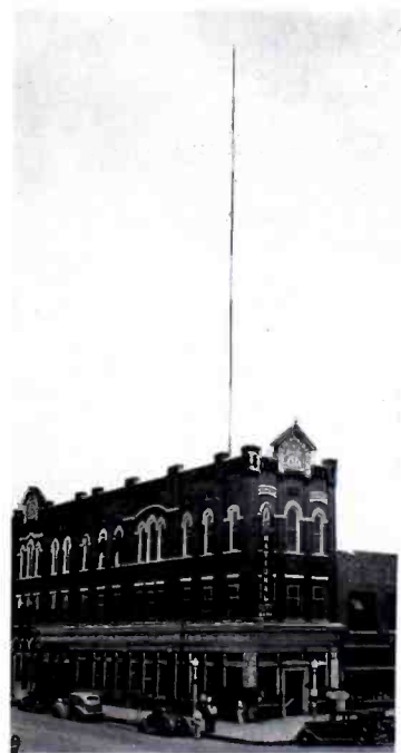
The new antenna at WRGA, Rome. An ideal type where it is necessary to place the antenna on the roof of a building.
