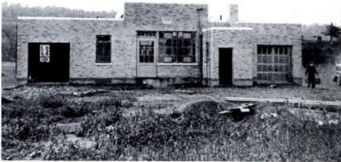
Rear view of WSYR under construction.
