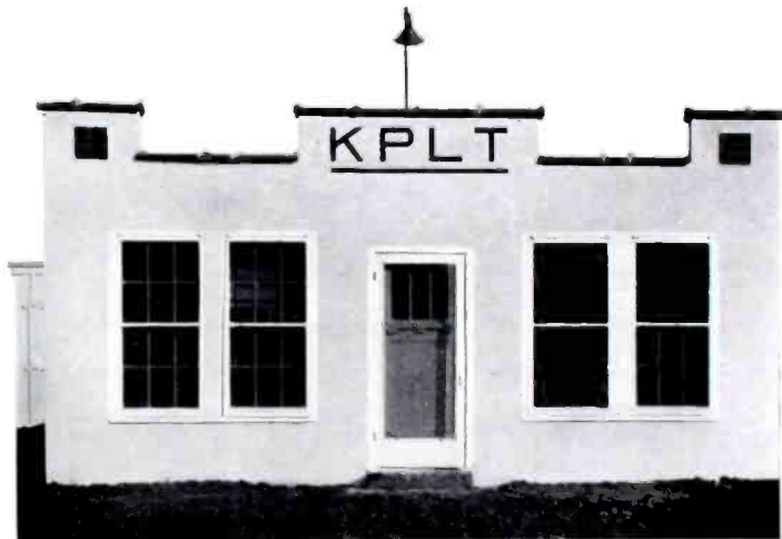
Front view of the new transmitter house for KPLT.
