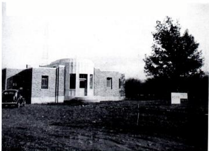
Front view of the structure before completion.
