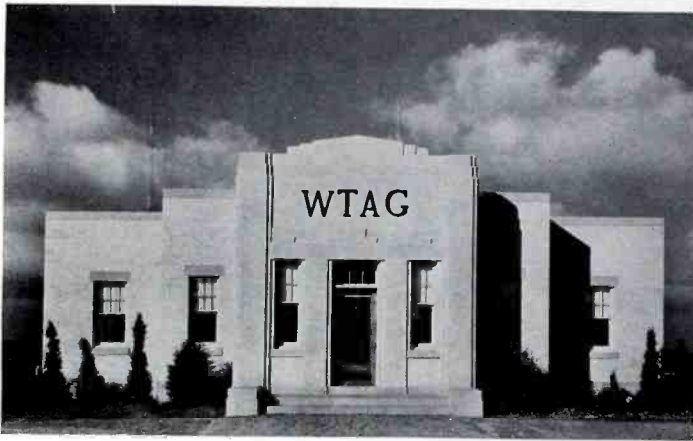
Completed home of important Massachusetts Station.
