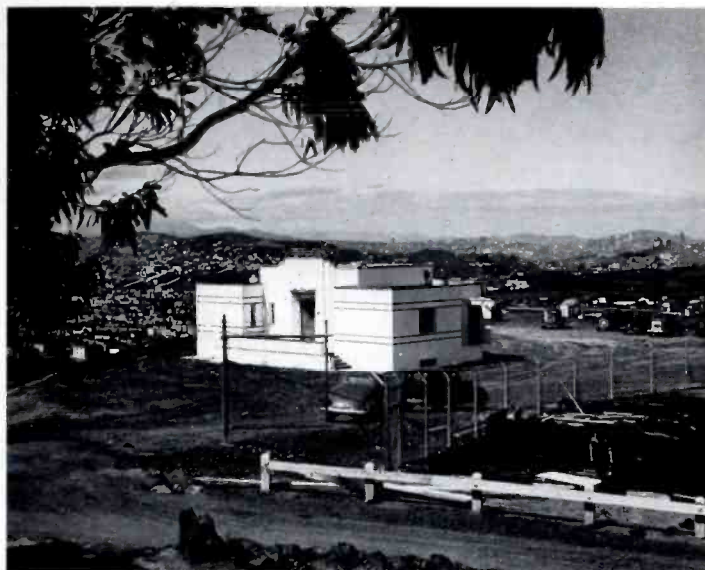
New transmitter house for KYA, San Francisco.
