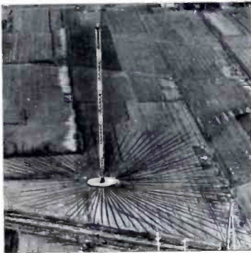
The new vertical radiator at WBEN with ground system converging at the base.
