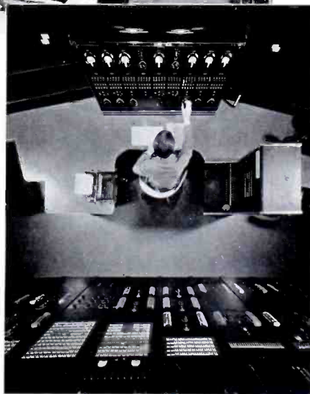
ABOVE: Transcription and Announcement Studio No. 6, showing 70-A turntable, 71-A vertical pickup, and 72-B recording attachment.
