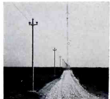
The transmission line for WLS looking towards the antenna.
