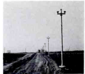
Looking away from the WLS antenna.
