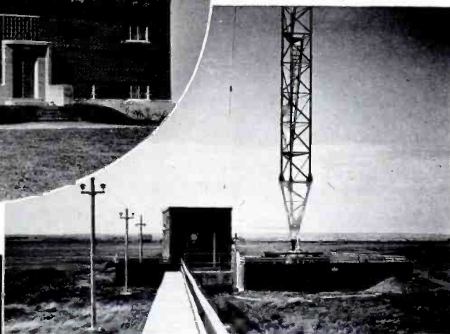
The CBA antenna coupling house and the base of the 460 ft. radiator.
