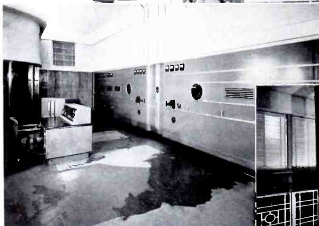
Above: RCA 50-D transmitter at CBK. The transmitter enclosure is finished in maroon.
