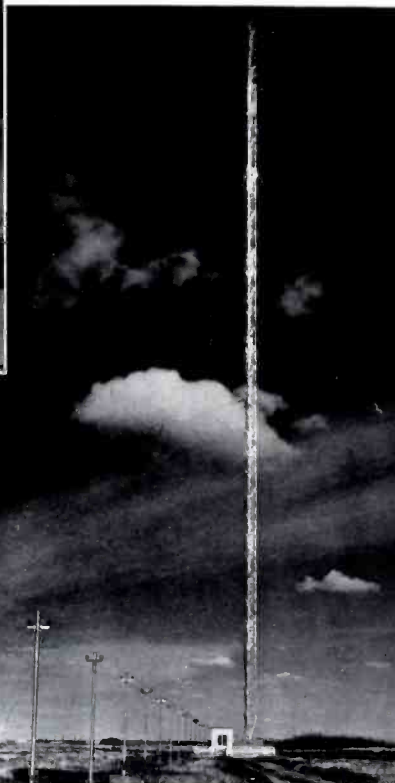
Above: 460 ft. Vertical Radiator and Transmission Line at CBK.
