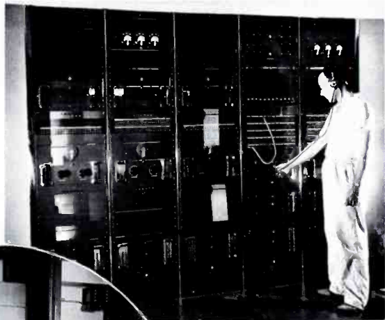
Above: Front view of the speech input racks with K. Sliker, Chief Engineer, doing the checking.
