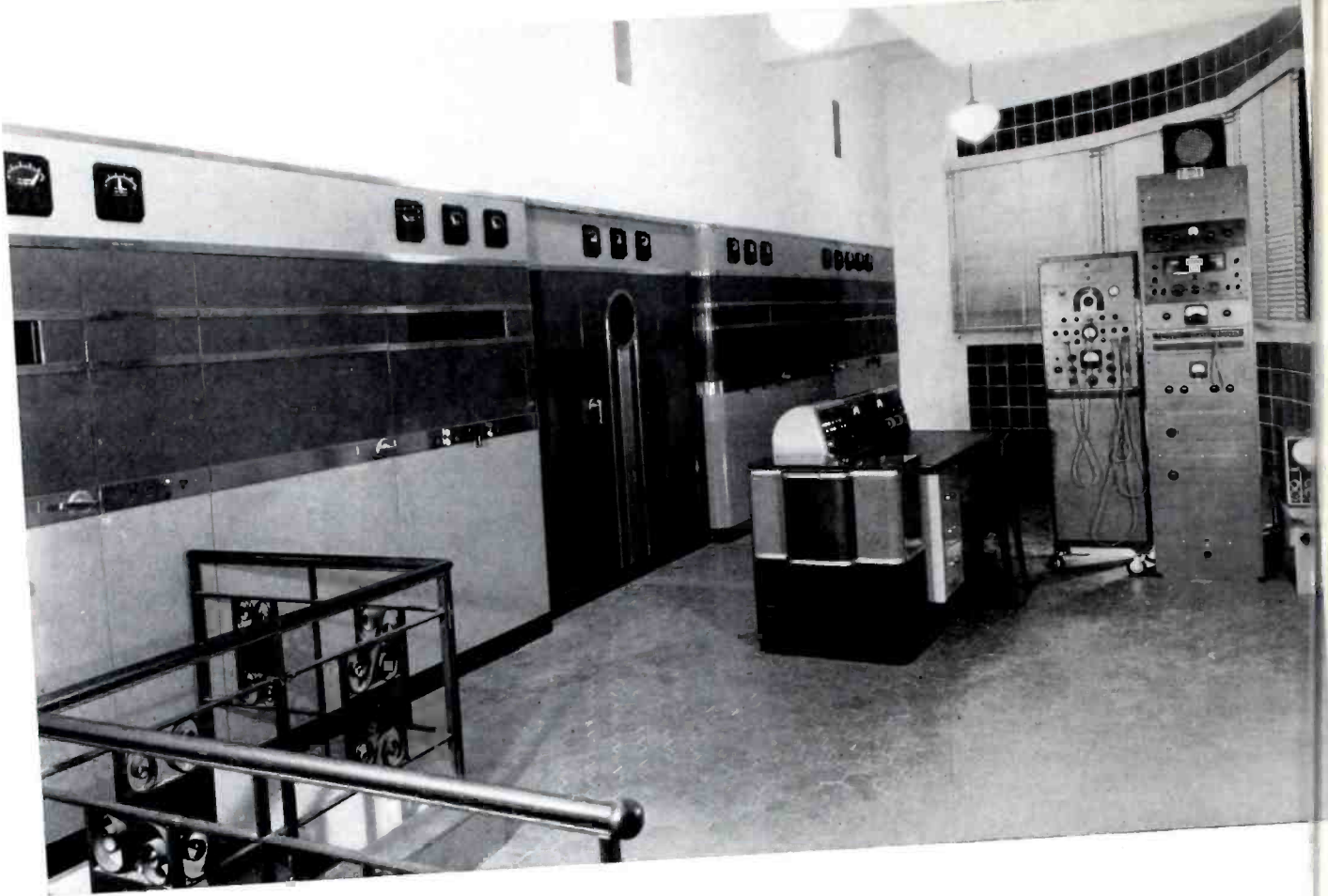
VOICE OF A GOOD NEIGHBOR —Front view of the RCA 50 KW transmitter at Radio Nacional with the console table, monitoring and measuring equipments, limiting amplifier, line amplifier and speech input equipment for emergency operations.
