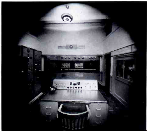
FIG. 1. 5-DX transmitter at WSYR, Syracuse. Cabinet for spare tubes and components is at the right; monitoring equipment and emergency transmitter at the left.
