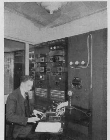
J. GULLENS ON DUTY BEFORE NO. 2 CONTROL ROOM APPARATUS AT REBUILT WJZ, OF THE NATIONAL BROADCASTING COMPANY AT BOUND BROOK, NEW JERSEY. THE OSCILLOGRAPH, ON THE RIGHT CENTER, IS USED TO MONITOR THE STATION OUTPUT. A MOTION PICTURE OF THE MUSIC OR SPEECH IS PROJECTED ON A REVOLVING MIRROR SHOWING ALL IMPORTANT DETAILS OF THE PERFORMANCE
