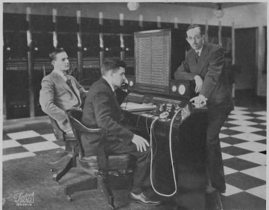
FIGURE 4—MASTER CONTROL DESK. AT RIGHT, O. B. HANSON, MANAGER OF NBC PLANT OPERATION AND ENGINEERING DEPARTMENT. AT LEFT, H. C. LUTTGENS, DIVISION ENGINEER. IN CENTER, J. C. MILLER, CONTROL ROOM SUPERVISOR
