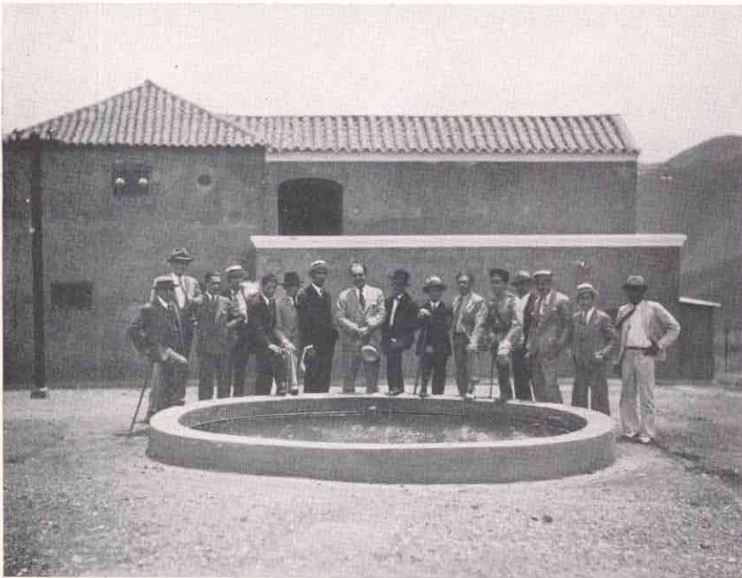
EXTERIOR OF THE STATION BUILDING, DURING A TOUR OF INSPECTION BY REPRESENTATIVES OF THE PRESS.
