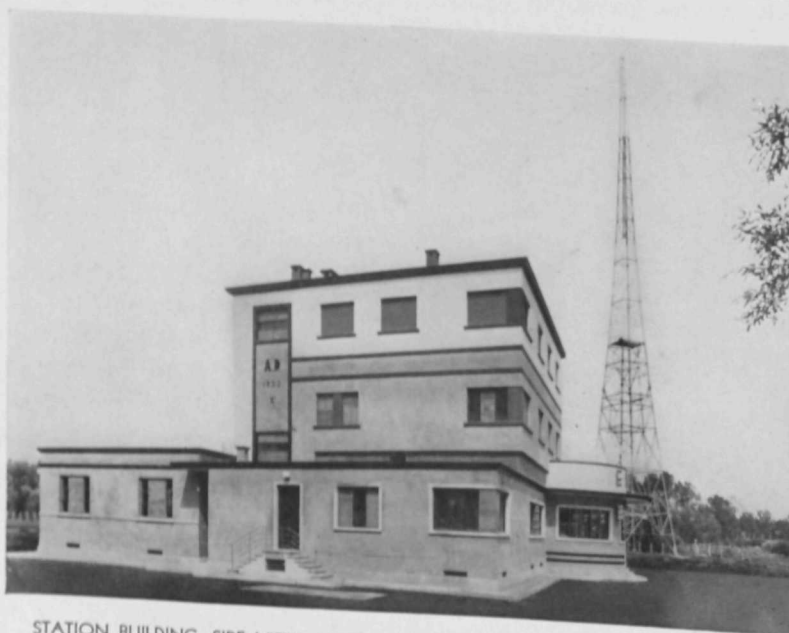
STATION BUILDING, SIDE VIEW—NOTE THAT BELOW THE INSCRIPTION "A. D. 1932" APPEARS "X," INDICATING YEAR TEN OF THE FASCIST REGIME.
