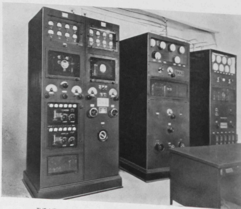
THE NEW 10 KILOWATT RCA TRANSMITTER EQUIPMENT AT WWL.
