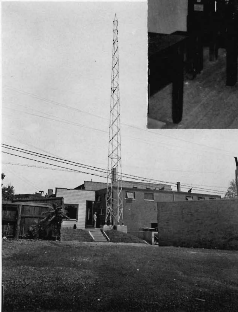
THE 94 FOOT BLAW KNOX VERTICAL RADIATOR OF WPFO, POLICE RADIO STATION AT KNOXVILLE, TENN. www.americanradiohistory.com
