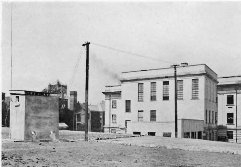
VIEW OF THE TRANSMISSION LINE AND "DOG HOUSE" AT LEXINGTON POLICE RADIO STATION, WPET.
