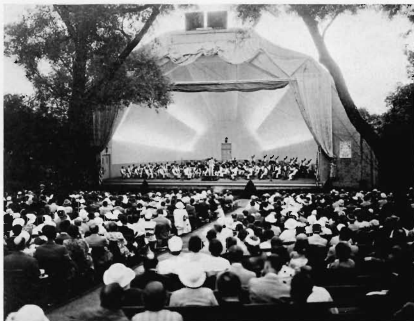
THE ACOUSTIC SHELL AT ROBIN HOOD DELL, FAIRMOUNT PARK. THE PHILADELPHIA ORCHESTRA MAY BE SEEN ON THE STAGE, AND THE TWO RCA VICTOR TEN FOOT DIRECTIVE BAFFLE LOUDSPEAKERS FOR SOUND REENFORCING MAY BE SEEN AT THE TOP OF THE SHELL. FOUR VELOCITY MICROPHONES MAY ALSO BE SEEN MOUNTED ON STANDARDS AT THE FRONT OF THE STAGE.
