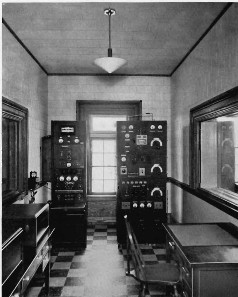
THE TRANSMITTER AND CONTROL ROOM AT STATION WGNY. ON THE LEFT IS THE RCA SPEECH INPUT RACK, WITH FREQUENCY MONITOR. ON THE RIGHT IS THE RCA 100 WATT TRANSMITTER. IN THE LEFT FOREGROUND ARE THE TWO RCA TRANSCRIPTION TURNTABLES. THE WINDOW ON THE LEFT AFFORDS A VIEW INTO THE LARGER OF THE TWO STUDIOS, AND THE WINDOW ON THE RIGHT AFFORDS A VIEW OF THE SMALLER STUDIO.
