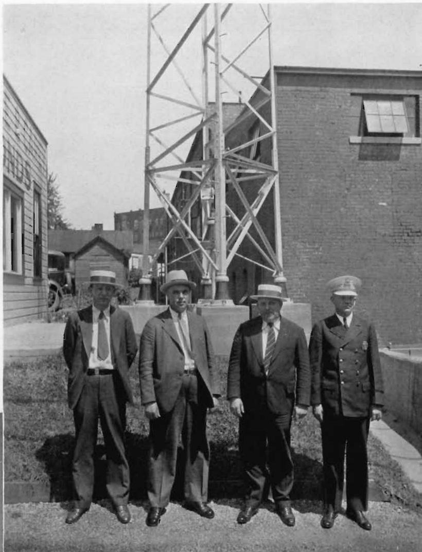
LEFT TO RIGHT—HAL H. HALE, CITY OFFICE ENGINEER, KNOXVILLE, SHERIFF BREWER, KNOX COUNTY, WALTER ANDERSON, DIRECTOR OF PUBLIC SAFETY, KNOXVILLE, AND CHIEF OF POLICE YORK, KNOXVILLE, OUTSIDE THE NEW POLICE RADIO TRANSMITTING STATION, WPFO
