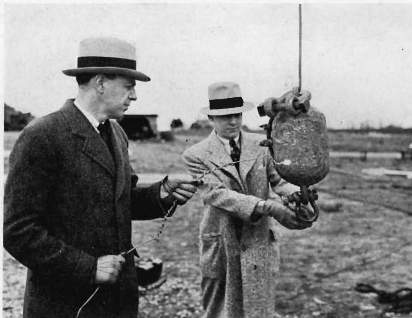
TOO "HOT" FOR COMFORT. LEW CROSLY, AT THE LEFT, OF THE CROSLY RADIO CORPORATION, AND J. A. CHAMBERS, TECHNICAL SUPERVISOR OF WLW, WSAI, AND W3XAL. THEY ARE SEEN DEMONSTRATING THE PHENOMENON OF RADIO FREQUENCY PICKUP AT THE WEIGHTED END OF THE CABLE HOIST USED IN CONSTRUCTING THE NEW WLW TOWER FOR THE RCA 500 KW INSTALLATION.
