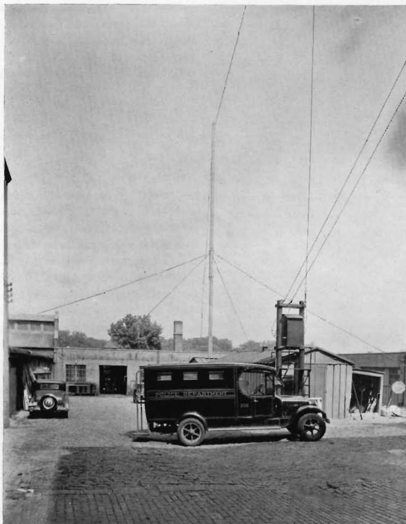
FIGURE 4—THE ANTENNA INSTALLATION AT WPFH, POLICE RADIO TRANSMITTER, BALTIMORE, MARYLAND.
