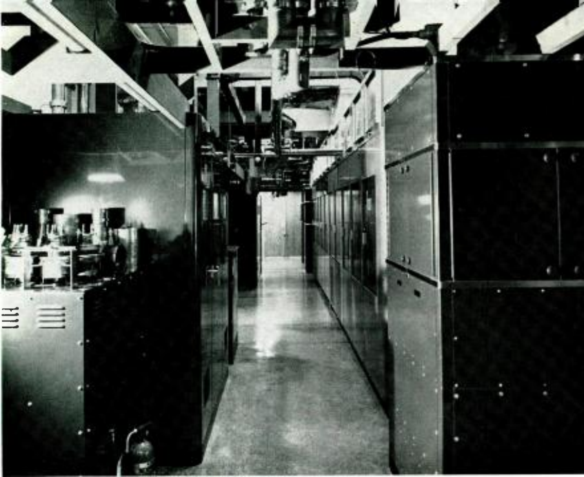
FIG. 9. Rear view of transmitter lineup. In this area all higher level coaxial lines and switches, dummy loads, sideband filters, diplexers, power combiners, high power rectifiers, transformers and switchgear have been installed.
