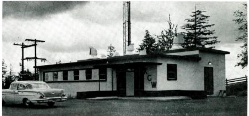
FIG. 5. The transmitter building is constructed of poured concrete and has 3200 square feet of floor space.
