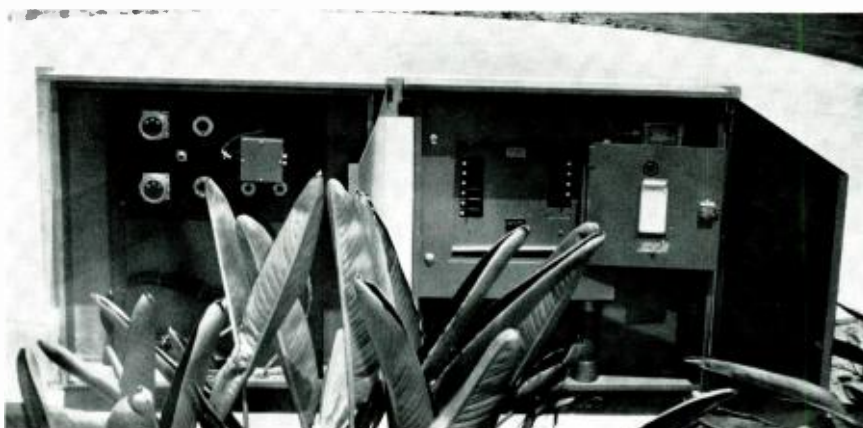
FIG. 15. Camera, microphone, intercom, and lighting outlet racks for outdoor shooting area.
