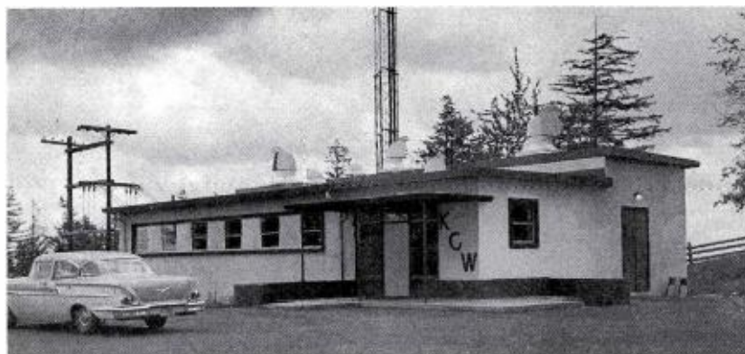
FIG. 5. The transmitter building is constructed of poured concrete and has 3200 square feet of floor space.
