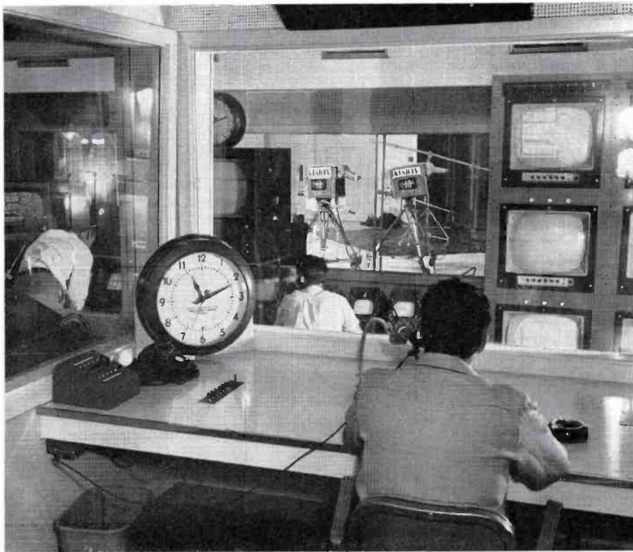
FIG. 8. Looking into Studio 2 from the Production Booth for this studio: to the left is the audio booth; in front is the video switching-control position. Production monitor rack is to the right. Note tally lights above monitors.
