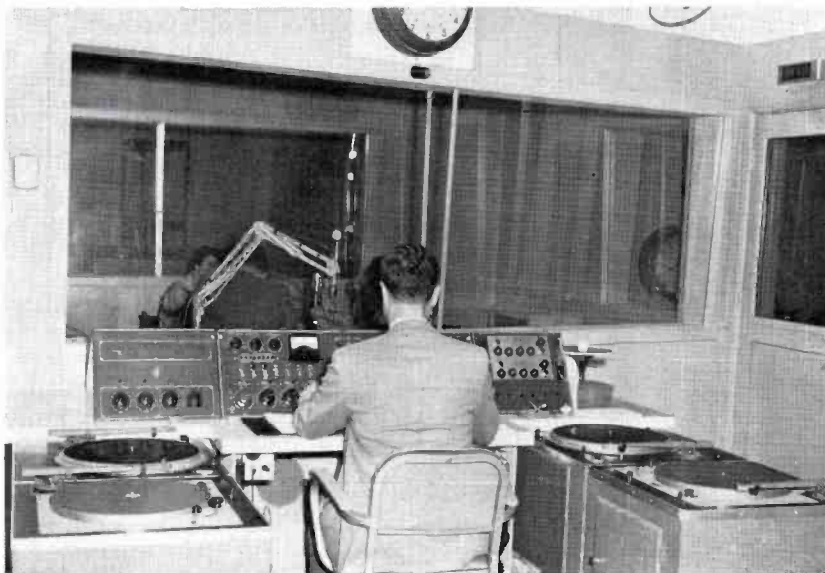
FIG. 19. Radio control position looking into radio station. Announce booth is to the right. In the background is control room of KFSD-FM.
