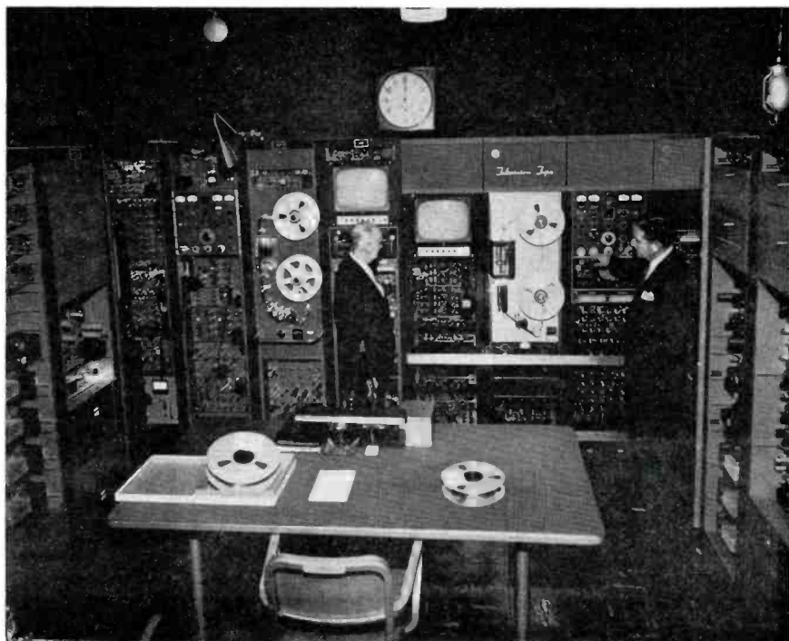
10:06 A.M. Last of the equipment racks are being set in place over trenches in the TV Tape area. The complete color tape recording facility includes (left to right) operations center (3 racks), color processing equipment (1 rack), auxiliary and power equipment (2 racks).
