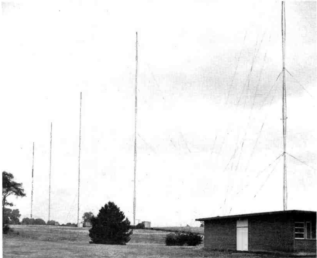
FIG. 11. Five in-line self-supporting towers are used in the WIBG antenna system. Small block houses at the base of each tower contain phasing and distribution equipment. The BFA type FM antenna is side-mounted near the top of the center tower.
