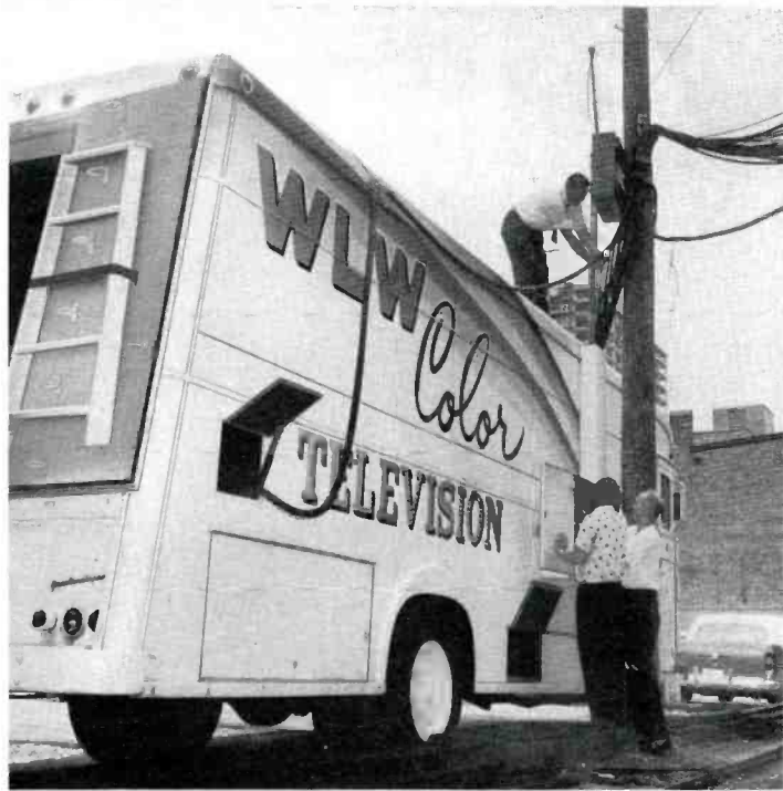
FIG. 12. Once the cameras have been stored in place in the mobile unit, cables are disconnected from the junction box on the side of the unit and hung in a weatherproof housing permanently installed on an adjacent pole.
