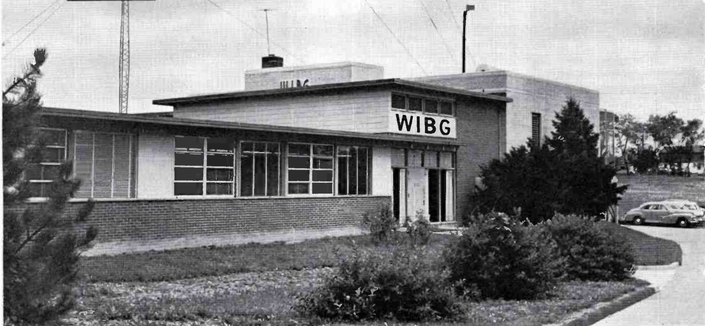
FIG. 1. WIBG's modern split level building located near Lafayette Hills in suburban Philadelphia shown here. The single story section (on the left) houses the station's offices. The larger section on the right contains the studios, control room, transmitter workshop, and garage.
