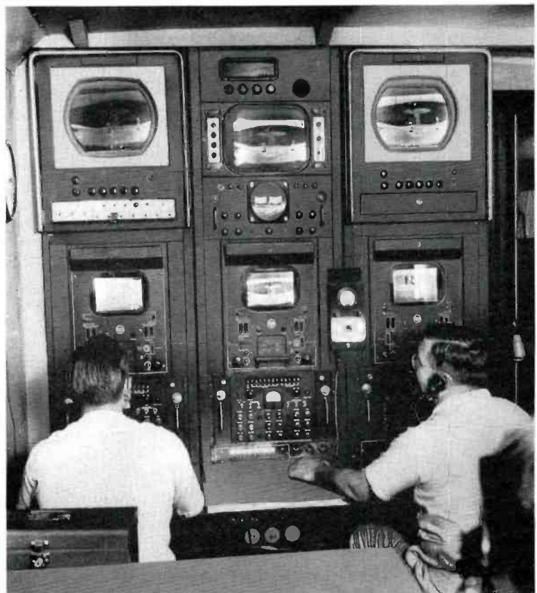
FIG. 5. Inside the mobile unit, two operators handle the controls for the three color cameras. Additional personnel on baseball remotes include an audio/video switching operator, a program director and a program commercial co-ordinator, all of whom sit on a raised platform overlooking the program monitors.
