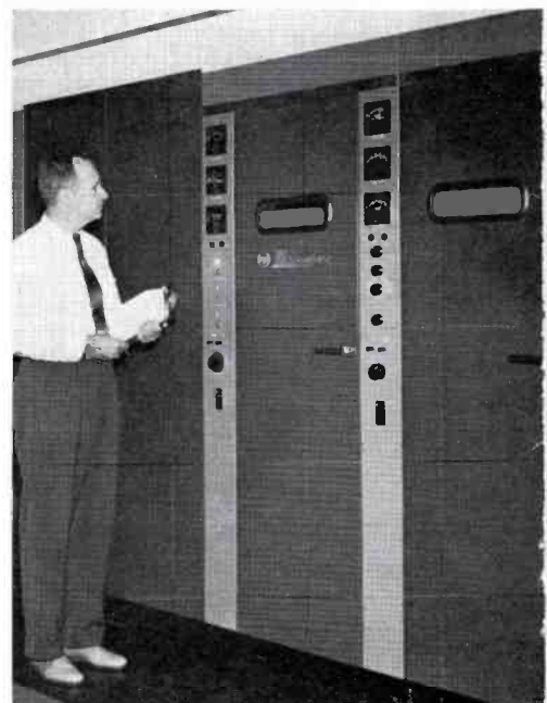
FIG. 7. The BTF-5B FM Transmitter is mounted along the rear wall of the control room. Lester Sacks is shown taking meter reading.
