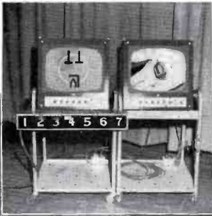
FIG. 5. In the classroom, students can ask questions and receive replies by means of a 2-way audio circuit. Inset shows monitors in studio—lighted number indicates question from classroom. Note microphone in student's hand.
