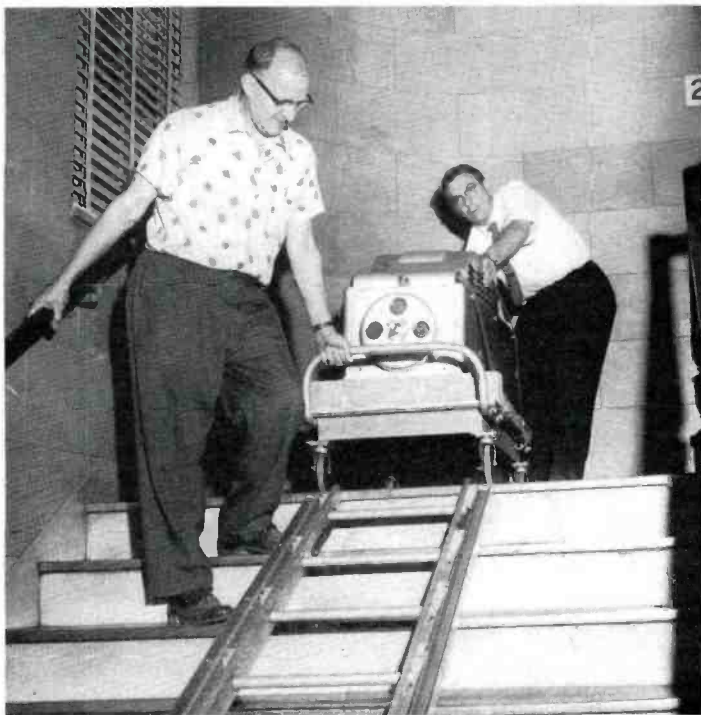
FIG. 11. The cameras are moved down a single flight of stairs to the alley aided by a specially designed aluminum track. This is essentially an aluminum ladder to which outside tracks are affixed.
