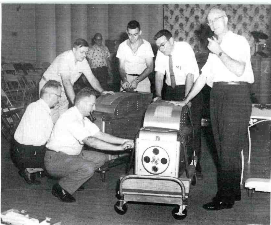
FIG. 10. The three RCA TK-41 Color Cameras are strapped to specially designed dollies to facilitate movement from the fourth-floor studio to the mobile unit parked outside the building. Camera pedestals remain in the studio, as tripods are used at the ballpark.
