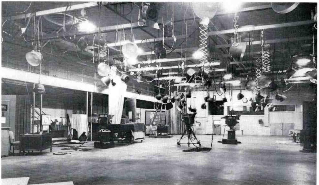
FIG. 4. WWL-TV studio. This 7000-square-foot area has three camera outlets at each of four stations. The one in the ceiling, shown here, has proven the most useful. Two trolleys bisect the studio to keep camera and microphone
