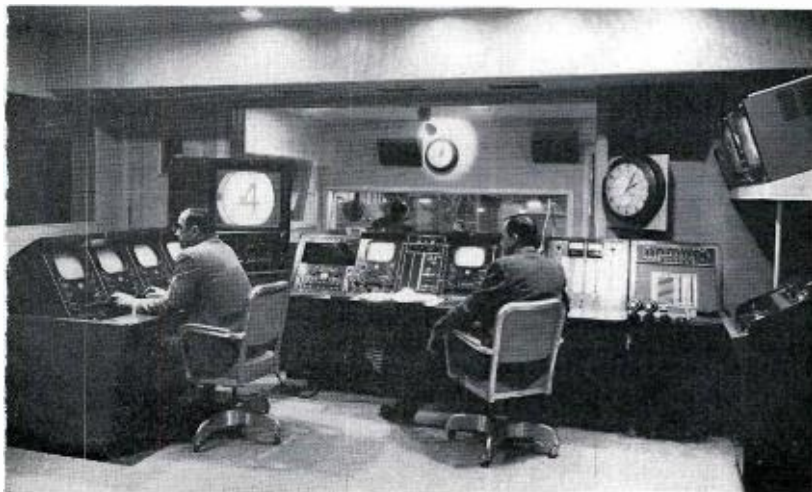
FIG. 9. Master control position with J. R. Lawton, Jr., master control supervisor, at video controls, and R. C. Warren at switching position. On the left are three TK-11 Camera Control Units, a TK-21 Control Unit, TM-21 Color Monitor, the TK-26 Controls and Master Monitor. At the switching position five consoles are used; the first, Remote Controls for two TA-21 AGC Amplifiers, a TA-9 stab amp, the TP-15 Multiplexer and variable density light filters. The next two house the preview and line TM-7 Master Monitors. The table in front of these units contains controls for the master control TS-21 Relay Switcher. In the fourth console is the master control audio switcher, designed and constructed by the WWL-TV Engineering Department. The fifth is used for telephone and intercom facilities with an audio tape recorder on the extreme right. The shelf (extreme right) has three monitors; one for network as received from telephone company, another microwave output, and the third "off-air" monitor. To the left of this area is the projection room and straight ahead is production control room with view of studio beyond.
