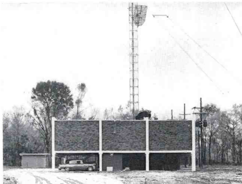
FIG. 16. WWL-TV Transmitter, near city of Gretna some five miles from downtown New Orleans studio, is housed in a modern brick and concrete building of windowless design. Unusual feature is placement of air circulating
