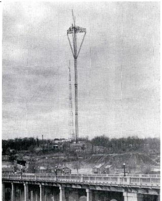
FIG. 15. The Candelabra is shown in contrast to the surrounding terrain. The overall height of the structure is approximately 1000 feet above sea level; however, the physical height of the structure is 730 feet.
