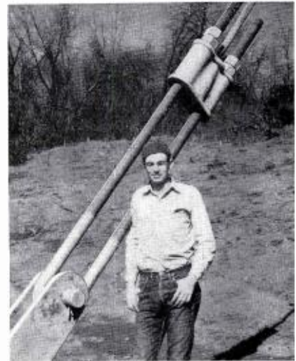
FIG. 6. One of the guy turnbuckles is shown in comparison to a man. (A dual guy system is used, making it easier to replace guy wires without jeopardizing the entire structure.)
