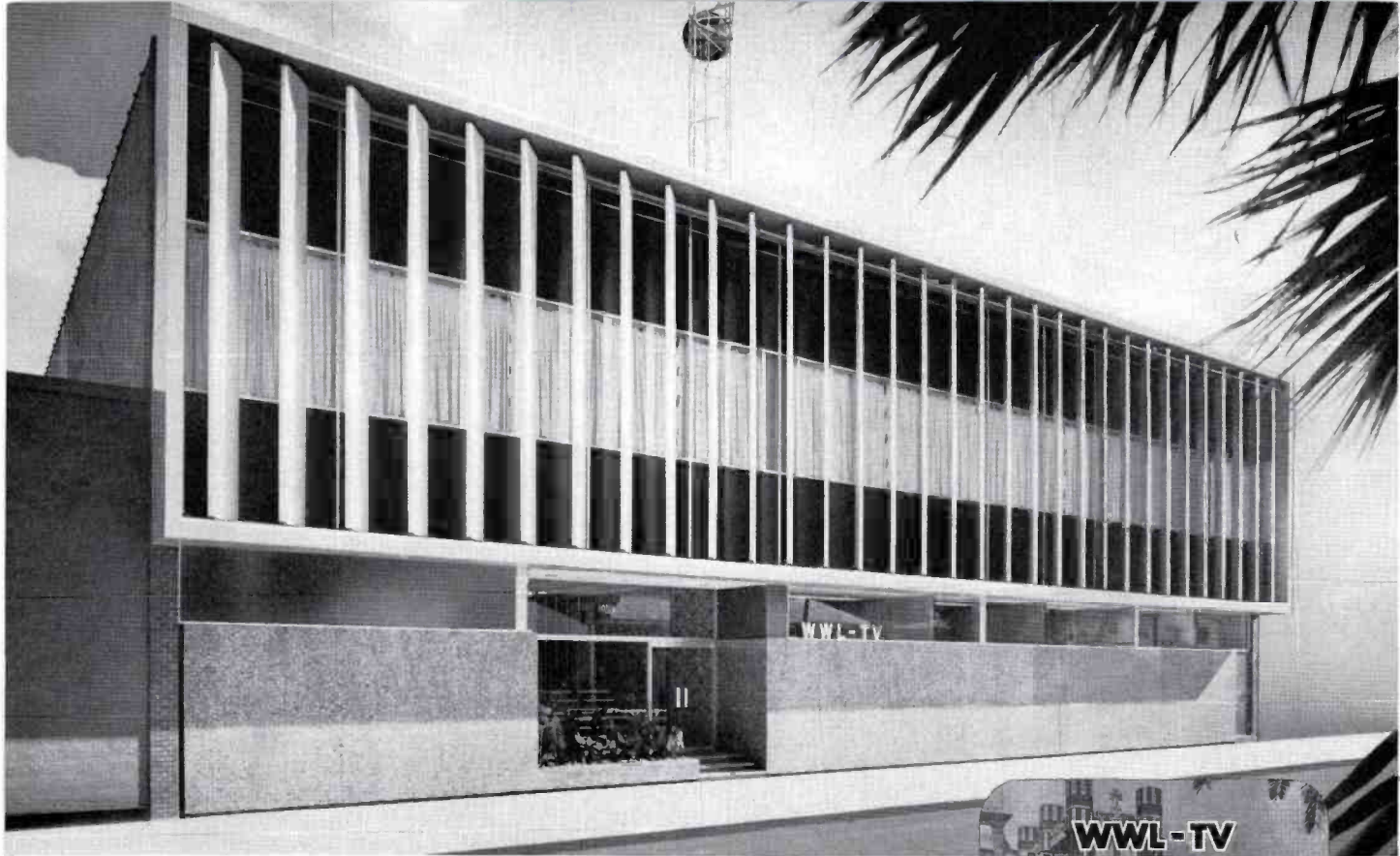
FIG. 1. Studio building of WWL-TV located in downtown New Orleans.
