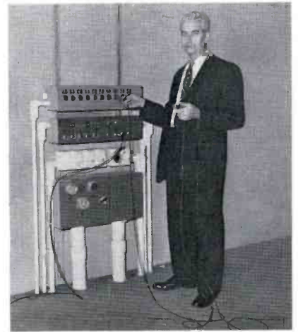
FIG. 3. Francis Jacob, Jr., chief engineer of audio facilities, at one of four termination panels in studio. Each contains 10 microphone, 9 audio and 2 video outlets; 2 intercom system, and 3 camera outlets. Conduit is in place for 3 more camera cables for color cameras.
