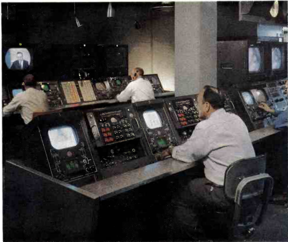
FIG. 2. Master and camera control areas are grouped for production efficiency. Control positions for all four color cameras face a line of color monitors at the front of the room. Master control with its custom built TS-40 Switcher is shown at the right.
