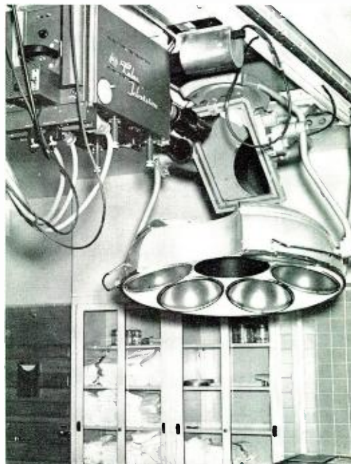
FIG. 3. U. of Mich. has surgical color TV camera installed in operating room of University Hospital.
