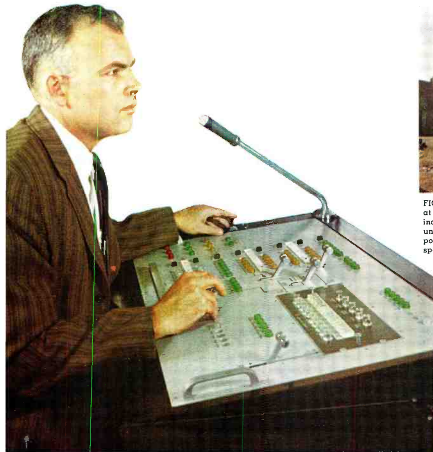
FIG. 4. Mr. Cobler, chief engineer, Skelton Studios, seated at technical director's desk in the production unit. It is here that "live editing" is achieved. The director can switch cameras, insert film and slides, and put special effects on tape—while the tv cameras are shooting the action.
