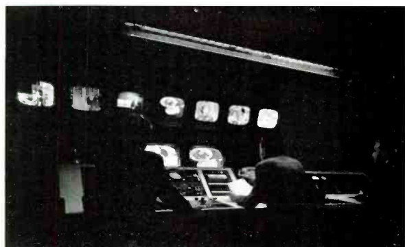
FIG. 1. This fully equipped tv film room facilitates film and slide inserts in color tapes. Color film to color tape transfers can also be handled.
