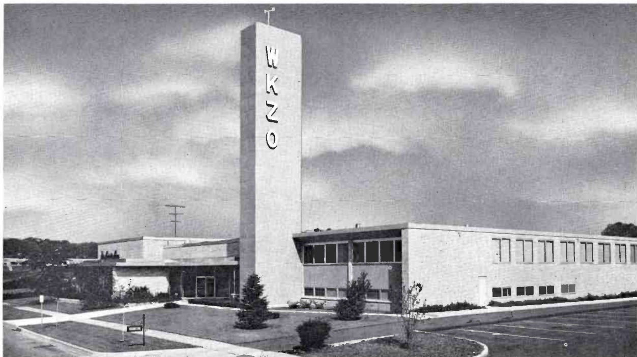
FIG. 2. Broadcast House. The 77-foot tower, at front, houses STL microwave and weather equipment. The building is of a tri-level contemporary design.
