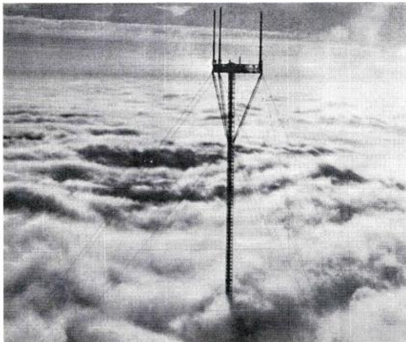
FIG. 10. The 1500-foot height of the candelabra often rises above a fog bank in the valley as shown in this dramatic photograph. The single structure, in spite of its height, is less of an air-traffic hazard than would be three separate towers.
