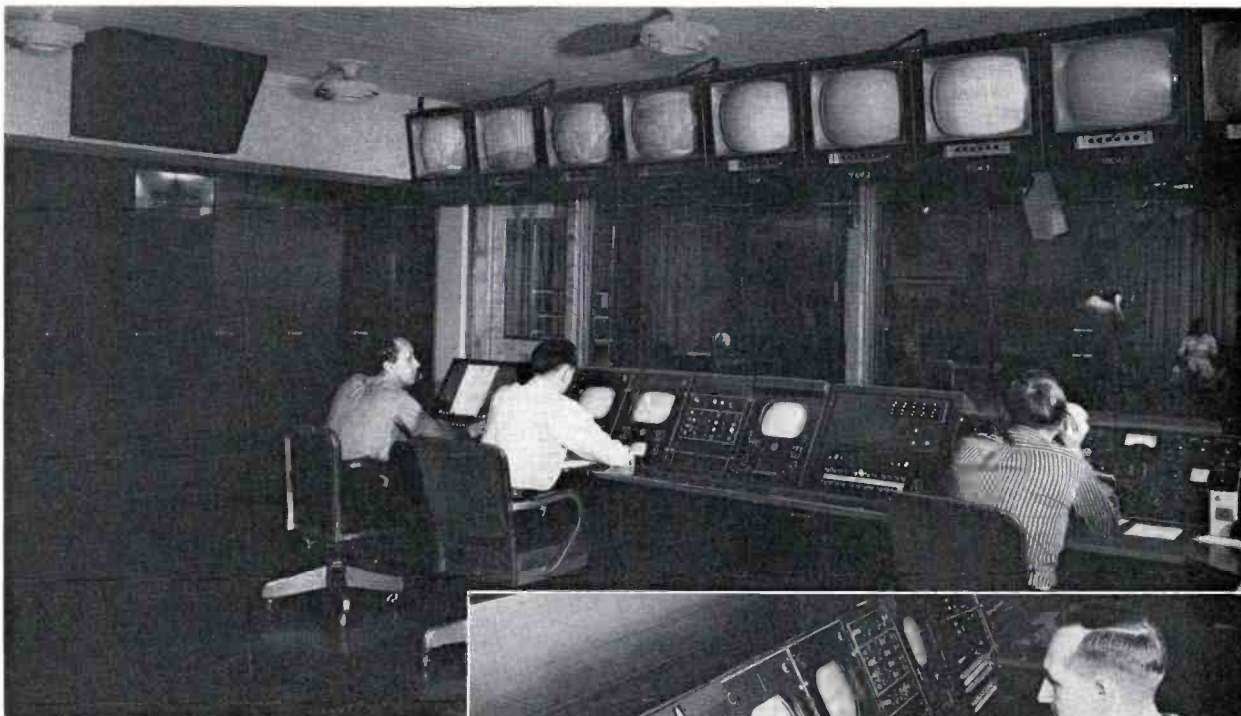
FIG. 8. WKZO-TV control room provides operators full view of "Studio 3", announce booth and film projection room.
