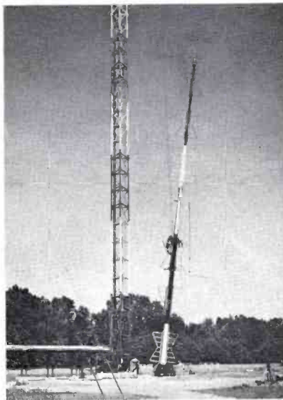
FIG. 17. Raising the top section of WKZO-TV's TF-12AL antenna.
