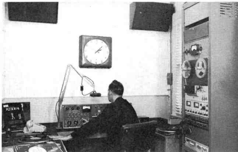
FIG. 8. All-RCA-equipped stereo-program center. BC-6B Audio Console at center, BK-5 announce mike on pantograph, BQ-51 turntables at announcer's elbows, RT-21 reel-to-reel tape deck and RT-7 cartridge facility mounted in rack at right, 12-inch studio speakers mounted on wall.
