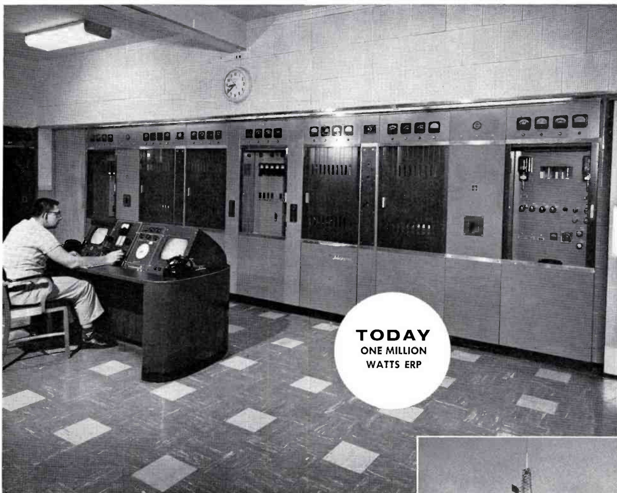
FIG. 2. TTU-25B UHF transmitter is the source of one million watts erp.
