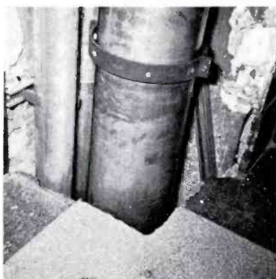
FIG. 5. (Upper Left) Vent shaft from 84th to 88th floors, used for transmission line. (Upper right) completing power changeover in transformer vault on 84th floor. (Lower Left) Installing TTU-50A Transmitter on 80th floor. (Lower Right) Transmission line and power conduit between 80th-84th floors. These were boxed in, plastered, and tiled.
