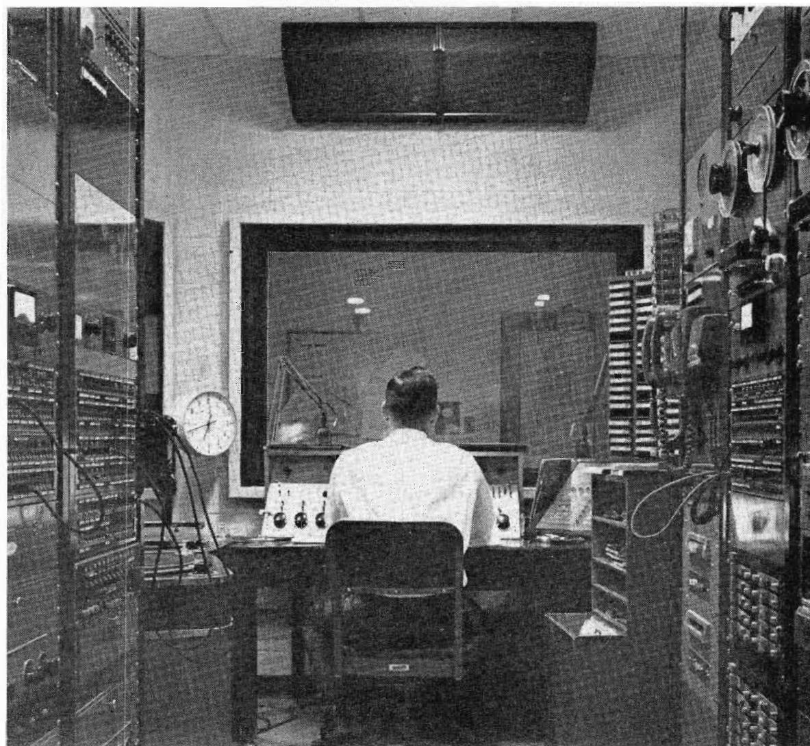
FIG. 29. Radio master control looking into Studio C.
