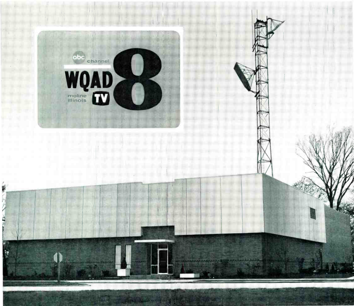
FIG. 1. WQAD-TV studio building, home of Moline Television Corp., Moline, Ill. On tower are Telco and station microwave reflectors. Programs are beamed to TV transmitter at Orion, Ill., 14 miles distant.
