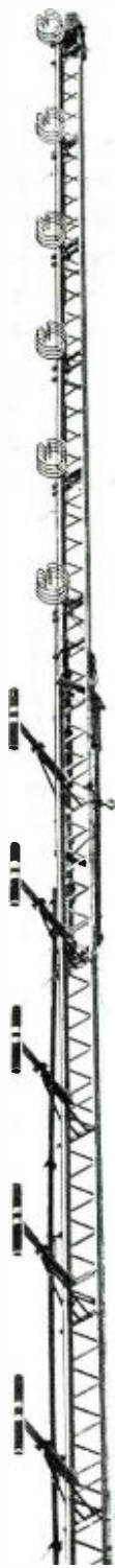
FIG. 2. The stacked "H" and "V" antennas of WSMJ (Greenfield, Ind.). Because of tower-loading considerations, the two antennas were stacked.
