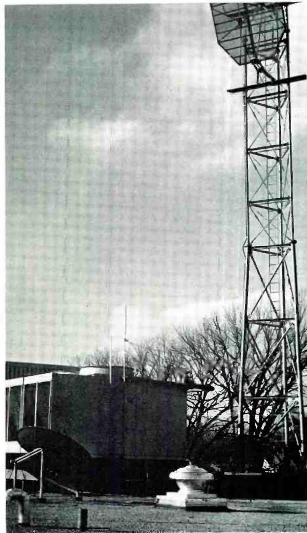
FIG. 25. On top of building is a 75-foot tower mounting reflectors for the microwave relays of the telephone company which bring network and other outside programs into WQAD-TV master control and the STL over which programs are transmitted from the studio to the transmitter.
