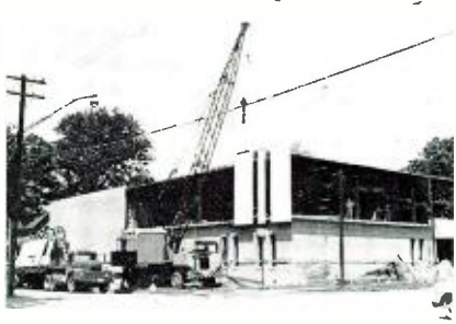
FIG. 4. Construction of new building started March 11, 1963 . . . by April 30 shell was erected and bricks laid . . . May 15 precast cement slabs arrived . . . During June and July equipment was installed . . . August 1 the station went on air!
