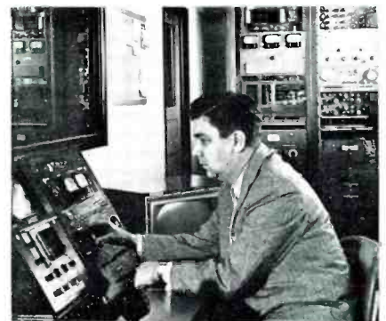
FIG. 26. Transmitter supervisor Bob Larson at transmitter control point, which also handles selection of diplexed microwave receivers.
