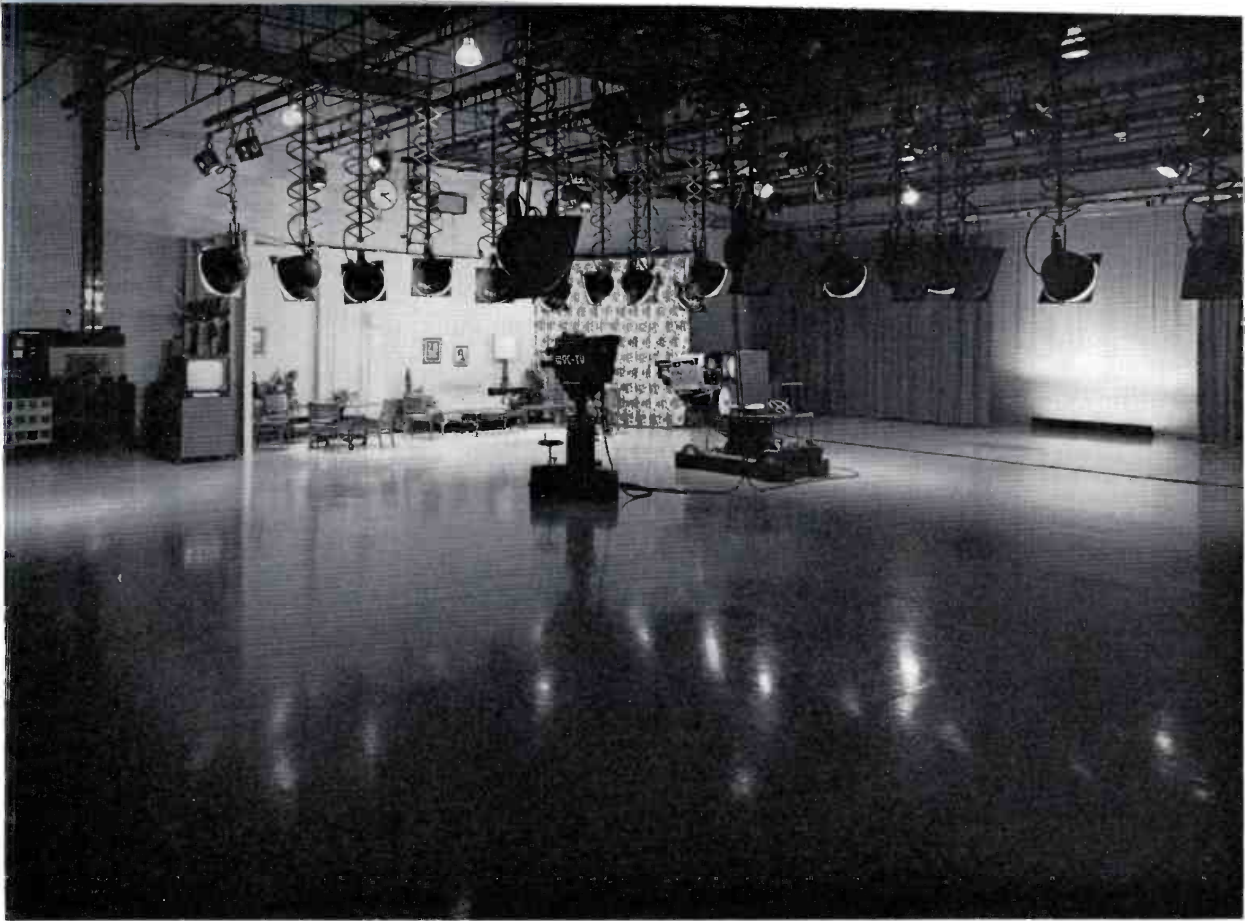
FIG. 3. Studio A, 2 stories high, more than 5000 sq. ft. in area, with 18-ft. turntable and newest RCA studio cameras is typical of modern facilities afforded by new WOC Broadcast Centre.
