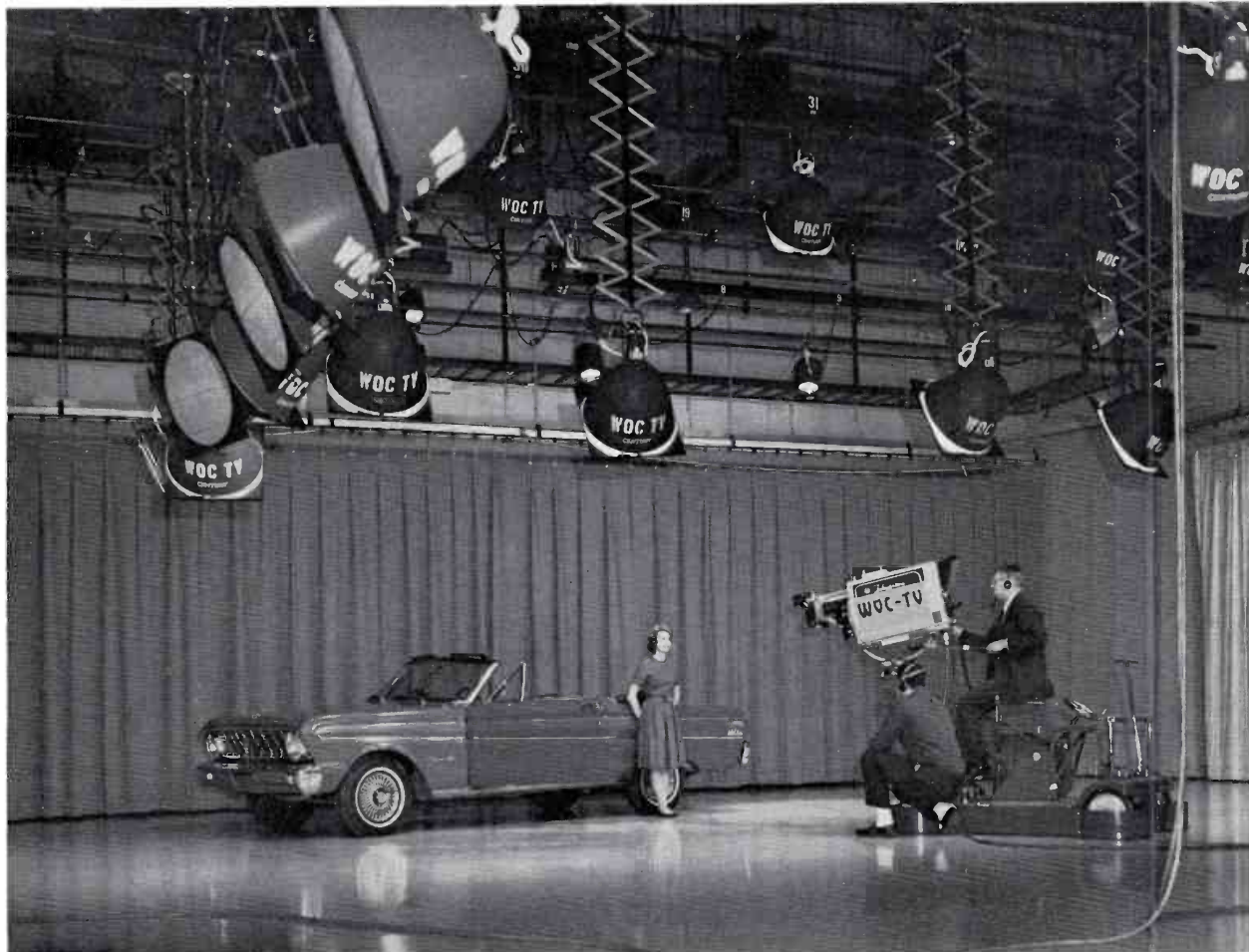
FIG. 29. Studio "A" includes 18-foot turntable with two mikes and a-c outlets. It will run up to 2½ rpm in either direction.
