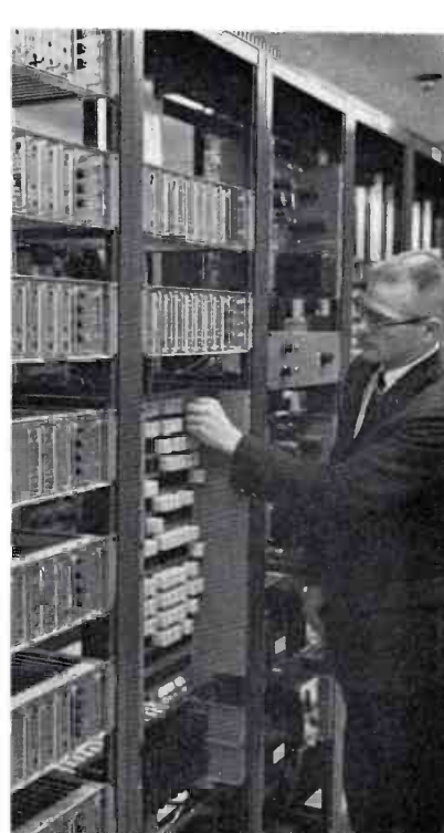
FIG. 32. WOC-built house monitoring system distributes 15 video sources to 15 offices and special areas. At left, are new RCA TA-24 Transistorized DA's (Pulse and video distribution system are completely solid-state.)
