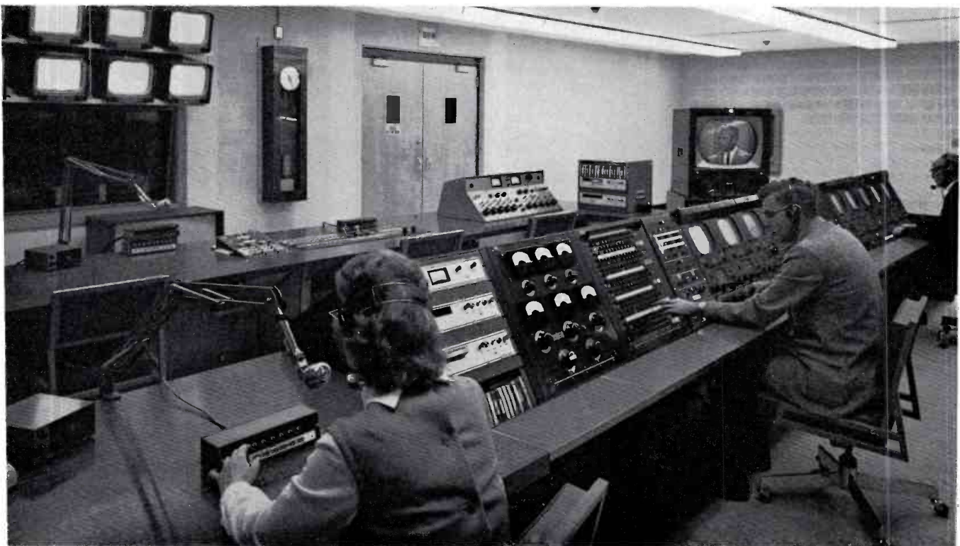
FIG. 24. Master Control in foreground, Studio "A" control in rear. Station breaks are handled at MC when "A" and "B" sub-controls are unmanned. All operations and switching can be done at MC when no live programming is going on.
