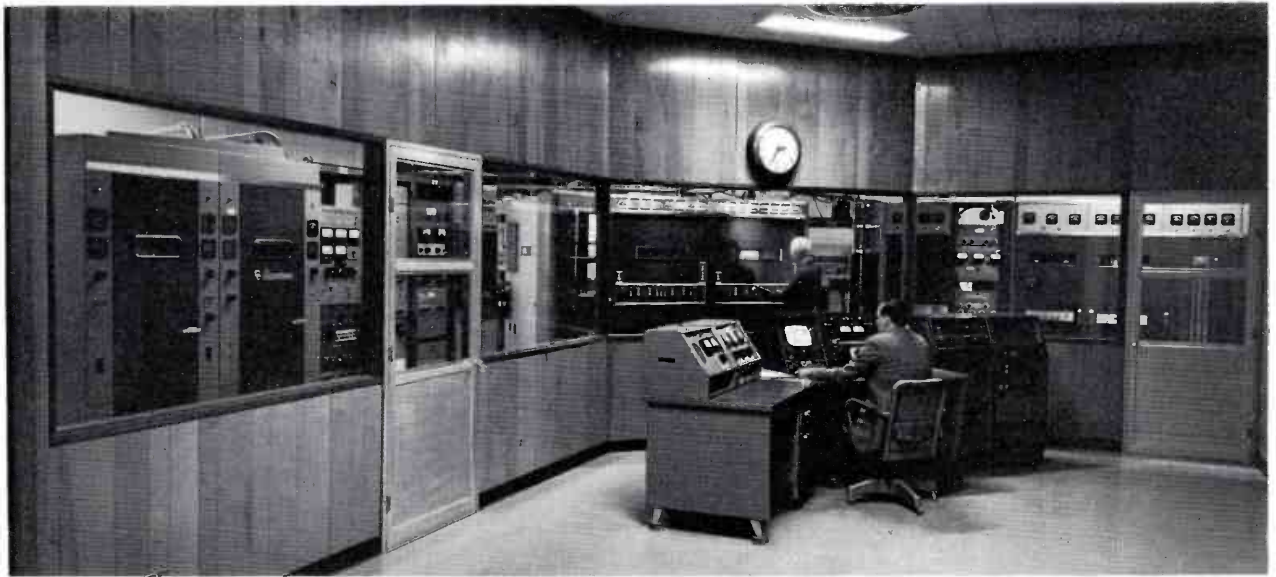
▲ FIG. 36. AM and FM Radio and TV transmitter installation. Radiating 100 KW on Channel 6. WOC produces highest signal strength in the area.
