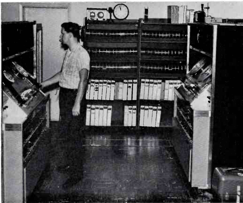
FIG. 18. TV Tape Room is located next to Projection and Master Control. Contains two RCA TR-22 TV tape recorders, with transistorized color modules. (A third TR-22 is installed in WFGA-TV mobile unit.) Recorders have remote start in Control "A", Projection, and Master Control.
