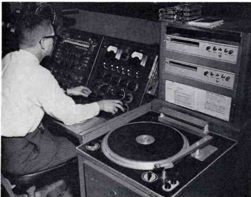
FIG. 22. Master Control Switching. Left panel contains video switching, stab amp controls, and remote start and stop switching for tape and projection equipment. Next panel contains audio program and monitoring equipment. Audio switching is normally interlocked with video, but an interlock defeat switch can lock any program source either in or out. Master Control can handle the air operation while other facilities are being used for TV taping or studio rehearsals.
