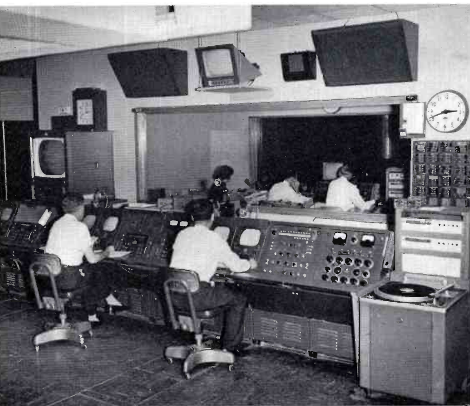
FIG. 21. In background is Control Room "A". Foreground (L. to R.): TK-11 controls; TK-41 color camera controls; TK-26 film color controls; master switchable monitor; master video switching panel; master audio switching panel; cartridge audio tape and RCA turntable.
