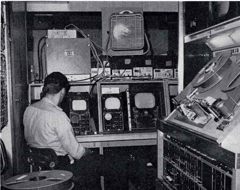
FIG. 25. TV Tape and transmission area in main mobile unit. Video patch, sync, and distribution amplifiers are located here.
