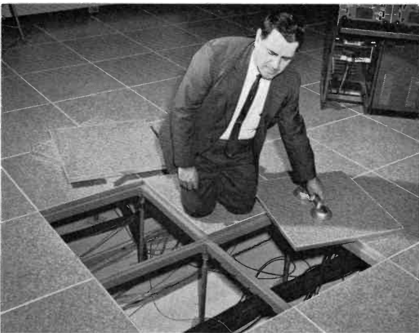
EASY ACCESS TO CABLING is a construction feature of the equipment room floor. A platform floor is elevated two feet above the floor level of Studios A and B. The photo above shows detail of its construction. A strut-like steel framework is supported at intersections by pipe stanchions (threaded for level adjustment). Over this frame are laid two-foot square blocks. The blocks are fabricated of \frac{3}{4} -inch plywood and steel sheets, topped with vinyl flooring, and encased in a frame of thin aluminum. Here a suction cup device (such as that used for handling large sections of plate glass) is being used to lift out the blocks for checking wiring between tape and film areas and the control console. These blocks form the entire equipment room floor. Use of this technique substantially expedited the initial installation of equipment. It also holds promise for ease of maintenance and simplified future expansion.
