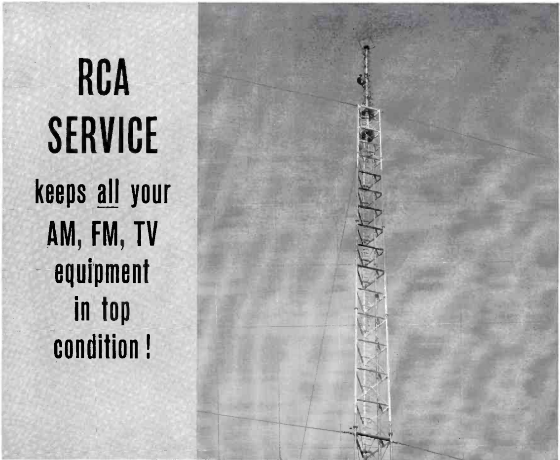
Antenna System Measurements
