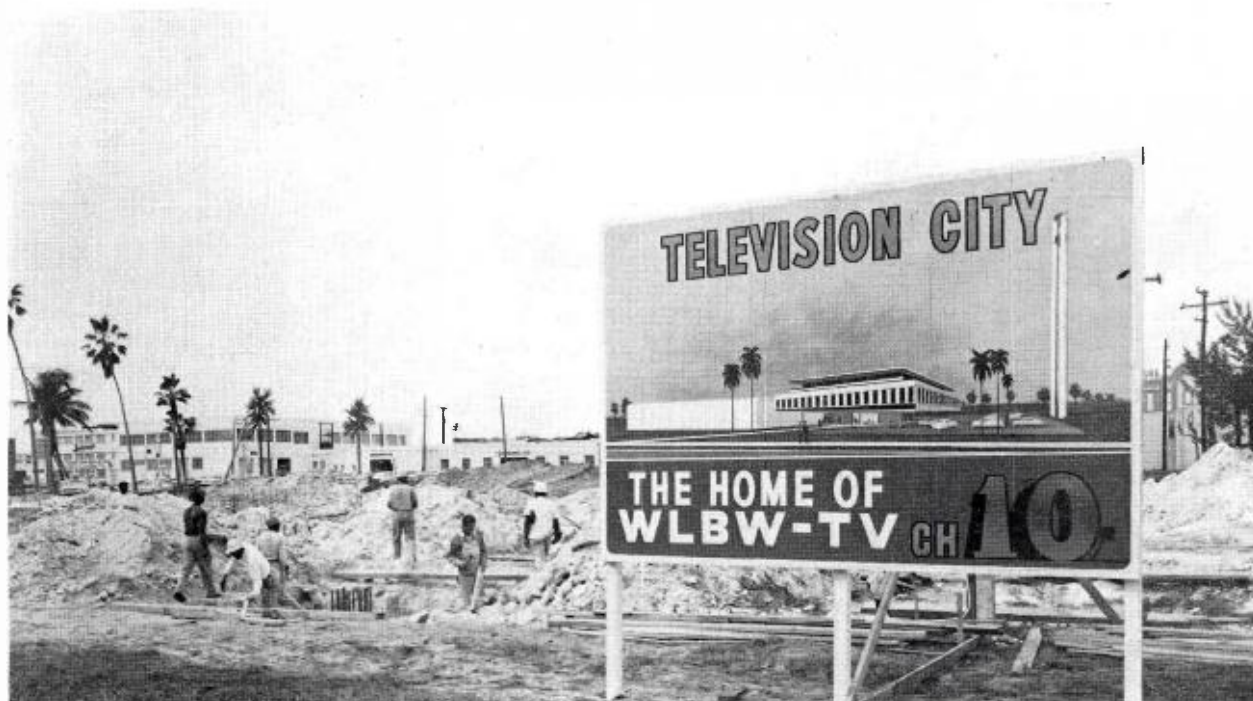
FIG. 1. Building site on Biscayne Boulevard for ultra-modern WLBW-TV Studios.
