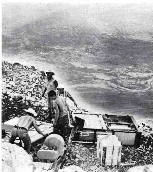
Work crew sorts pay loads of several flights as assembly job begins.
