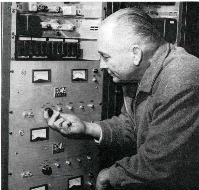
FIG. 3. A portion of the RCA 2500 MHz transmitter equipment installed at the Communications Center at St. Joseph's Seminary in Yonkers, New York a part of the Archdiocese of New York ITV System.
