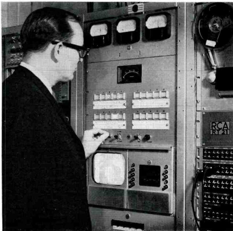
FIG. 2. The WKBS remote control rack installed in the Studio Master Control Room. E. R. Hill, Director of Engineering for Kaiser Broadcasting is shown operating the RCA BTR-20C Remote Control Studio Unit.
