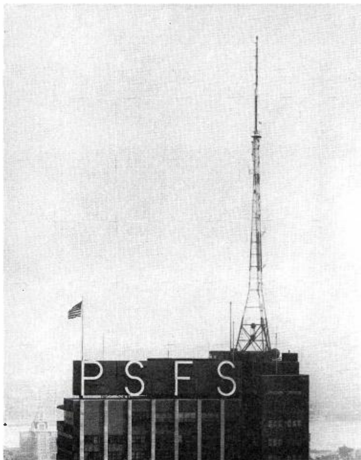
FIG. 1. BFC-4 Circularly Polarized Antenna of WMMR-FM, Philadelphia.
