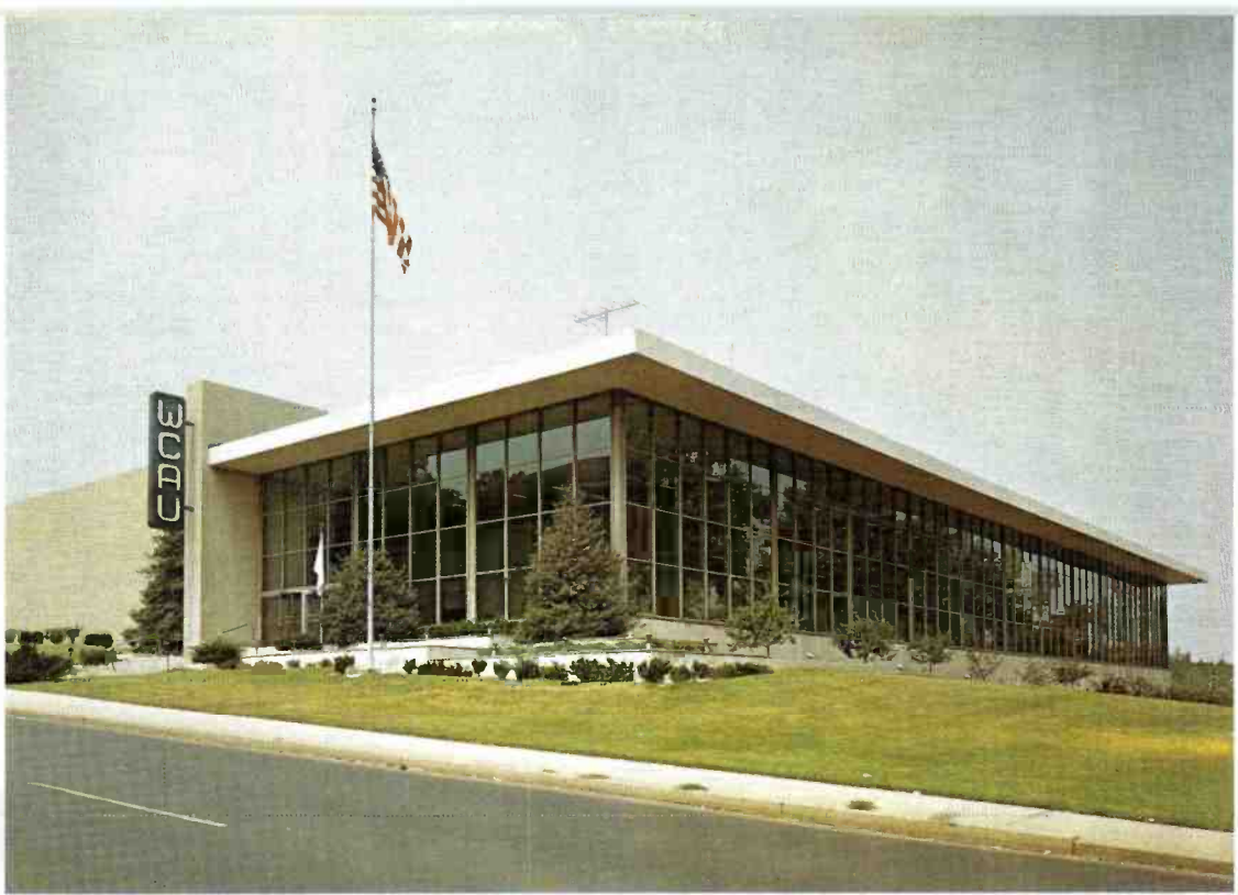
FIG. 1 At City and Monument Avenues in the Philadelphia area, the WCAU-TV building houses a most modern television broadcast center.
