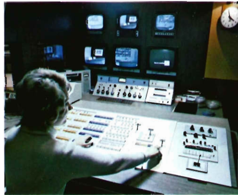
Other production facilities get full-time utilization in completely equipped "Studio 12".
