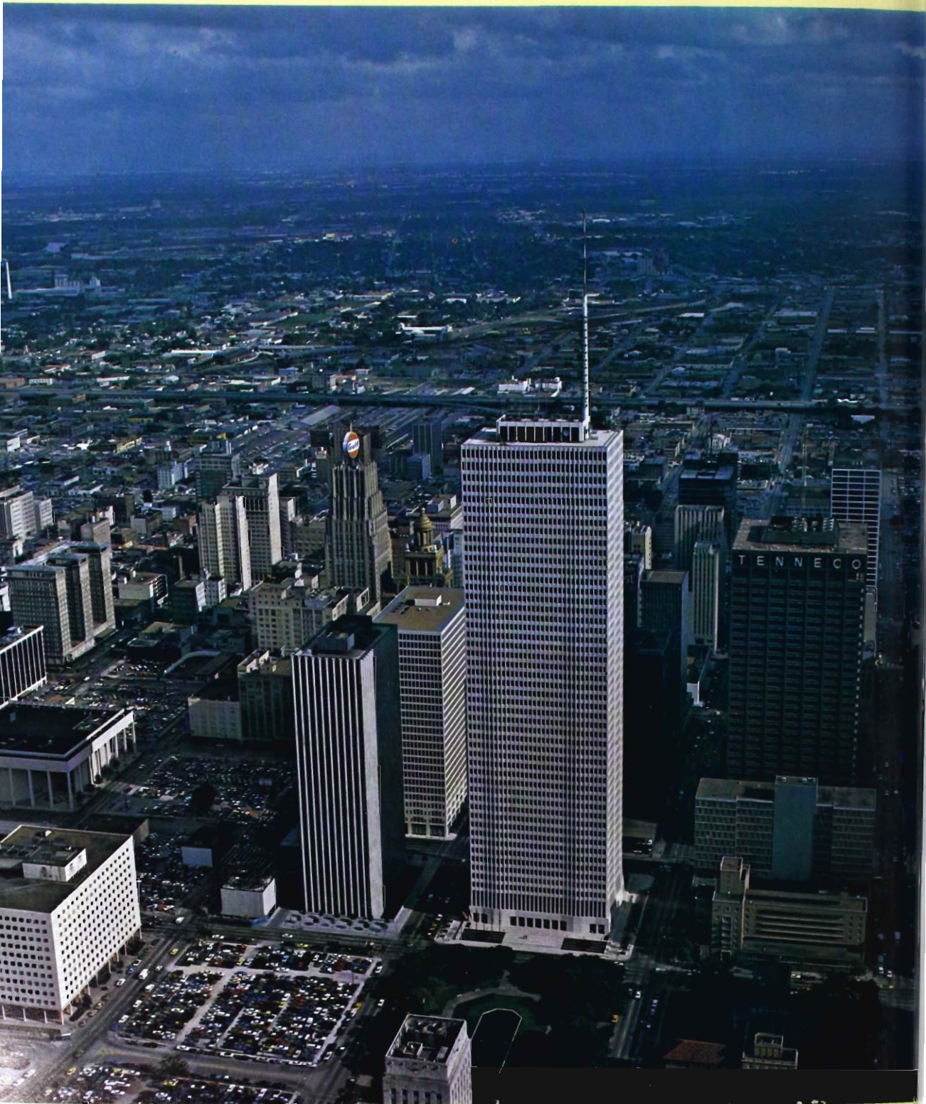
KVRL's omnidirectional antenna atop One Shell Plaza in downtown Houston covers the city with a clear, unobstructed TV signal.
