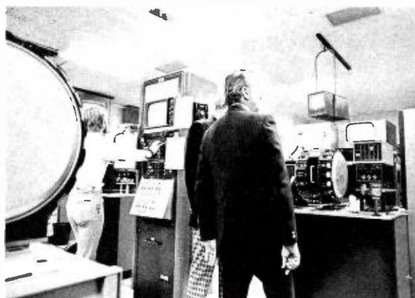
In the Film Room, machine controls for the four TK-27 film systems are remote to a central panel. A second set of remote panels is in Master Control.
