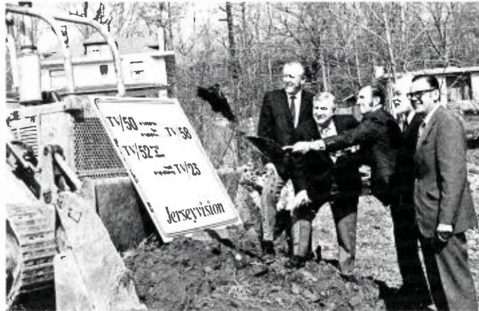
Wielding the shovel for this distinguished groundbreaking crew is Dr. Edward J. Meade, Jr., Chairman of the New Jersey Public Broadcasting Authority. Other participants include (left to right) John Wilner, Director of Engineering; Maurice M. Veneri, NJPBA member; Henry P. Becton, NJPBA member; and Dr. Lawrence T. Frymire, Executive Director.
