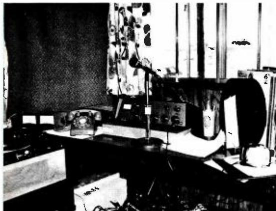
New broadcast facility for KRXX-AM is installed in a mobile home. Temporary studio set-up includes the basics for broadcast operation.
