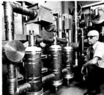
Chief Engineer Don Ferguson shown with filterplexer for TT-35FH. The Ch. 10 transmitter is manned only part-time for handling routine maintenance.
