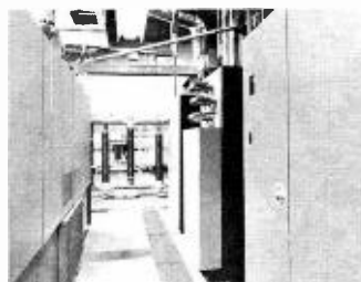
Front and rear view of KCRA's TT-30FL transmitter system. Remote control rack faces transmitter to facilitate making on-site test checks.
