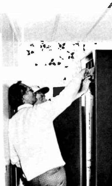
Station owner Don Ellis (below) checks out the RCA BTA-1S transmitter which replaced the bathtub in the mobile home.
