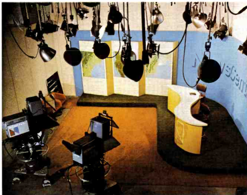
Main Studio with News set. is also used for production. Hydraulic lift covered by rug permits bringing up props from basement storage area.
