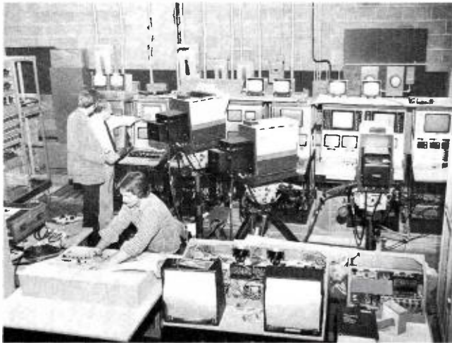
Space is available in the CRAE Shop for wiring, assembly and test of complete systems before shipment to customer installation site.
