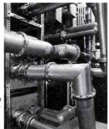
Transfer panel at WITF-TV. Manual patch panel at left; motorized coaxial switches on right.
