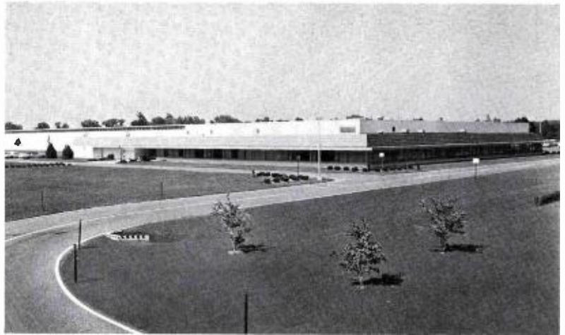
Extensive electronic parts depot at Deptford, N. J. stocks more than 48,000 different broadcast equipment parts.
