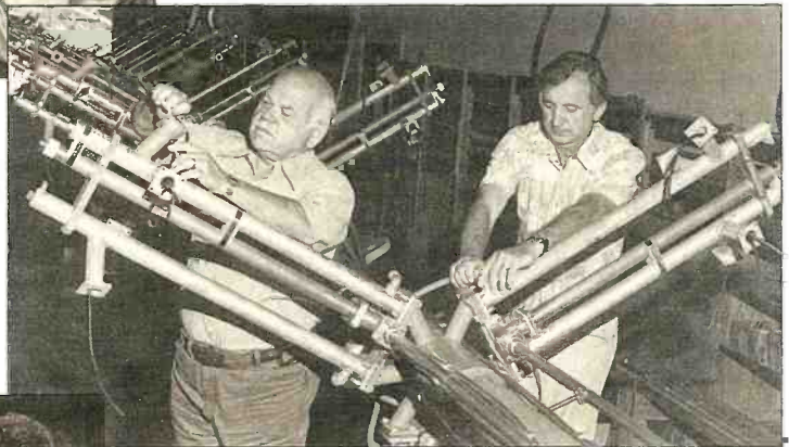
Wiremen at work on antenna inside one of the two assembly buildings (right).
