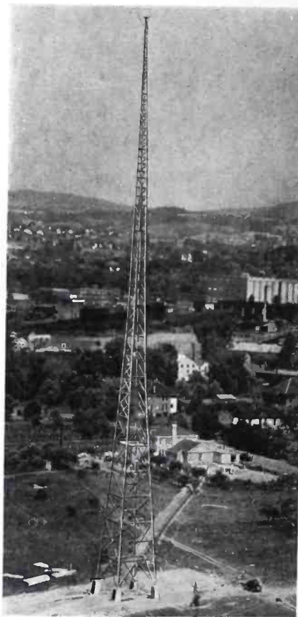
Looking over the city from the antenna site.
