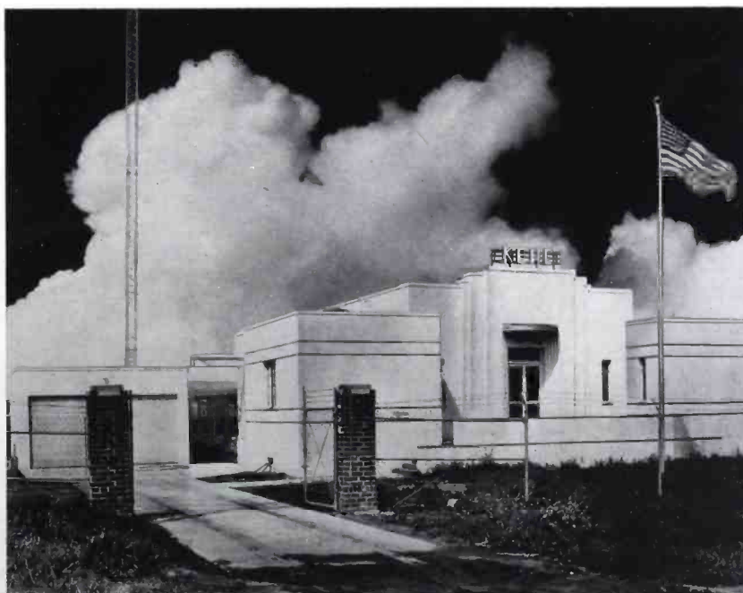
The new transmitter house, also modernistic in design.
