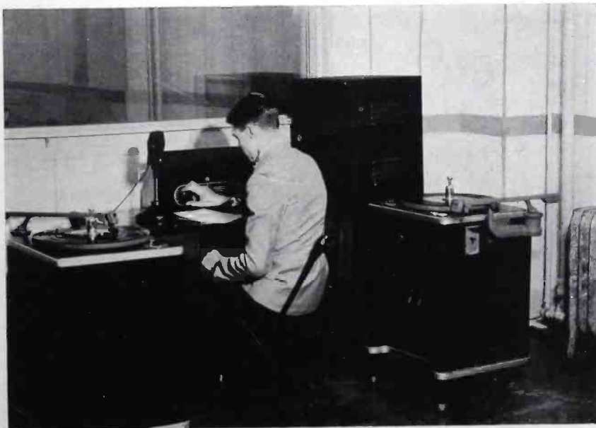
Transcription equipment in control room.
