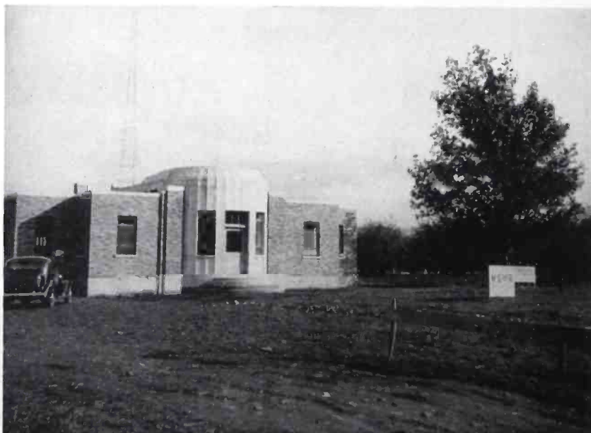
Front view of the structure before completion.
