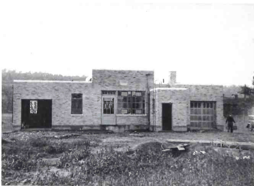
Rear view of WSYR under construction.
