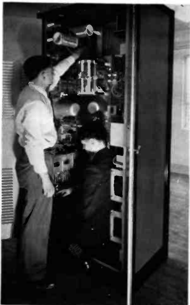
At WMBO in Auburn, New York, the 250-D is set up and connected to external wiring. RCA's Engineer, James Keachie assists Herbert J. House of WMBO in the final adjustments.
