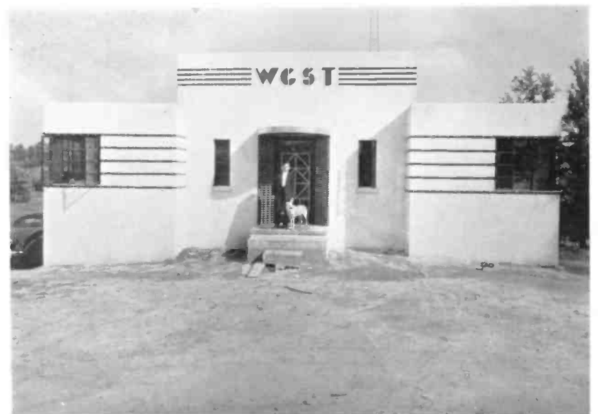
Above, WGST is decidedly modernistic in the construction of its transmitter house.
