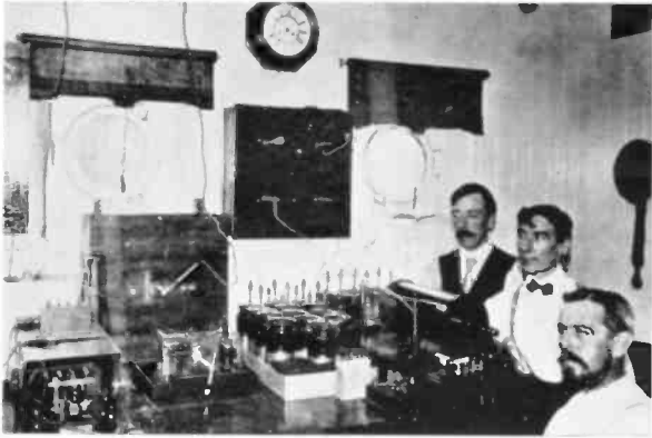
An 1897 radio station complete with spark coil and coherer detectors.
