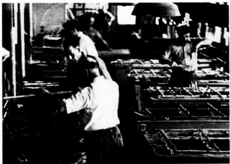
14. Rust protection is important. Frames, metal panels, shields, all are rust-proofed before applying final finish. Here in the copper plating shop, components are receiving a protective coating.
