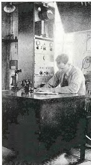
A corner of the control room.
