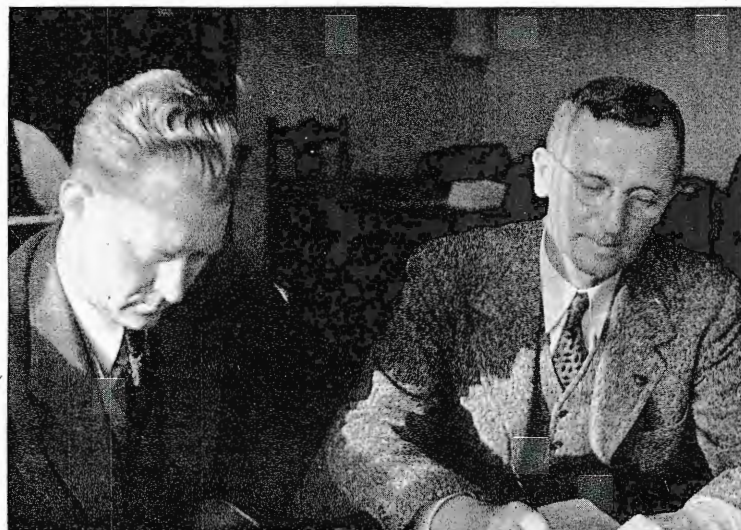
Messrs. J. C. Bell, Secretary-Treasurer, and K. G. Marshall, Vice-President, Birmingham Broadcasting Corporation, signing the order for the RCA 5-D transmitter now in operation at WBRC, Birmingham, Alabama.
