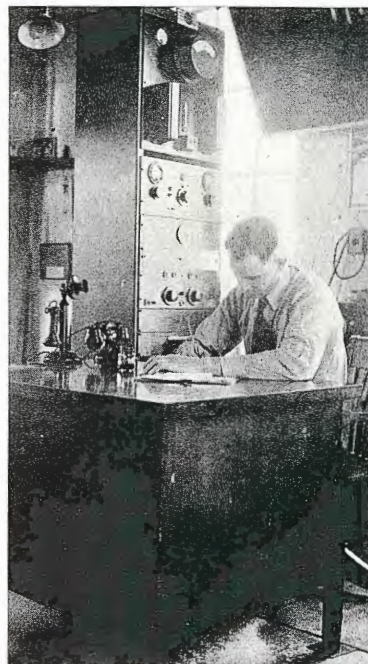
A corner of the control room.
