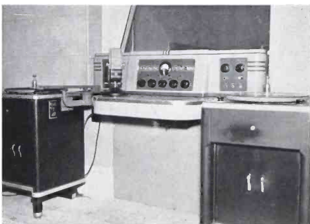
◀ Studio Control Room.
