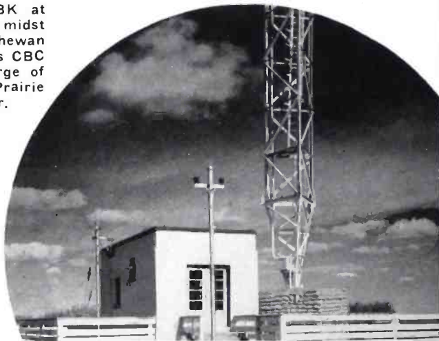
Antenna Coupling house at the base of the CBK Radiator.
