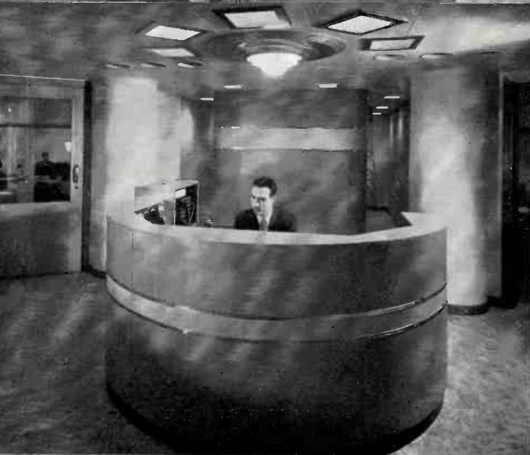
FIG. 2. (Center left) Another view of the master control desk. The equipment room can be seen directly behind the operator. The equipment is completely enclosed behind and is "pressurized" with filtered, refrigerated air.
