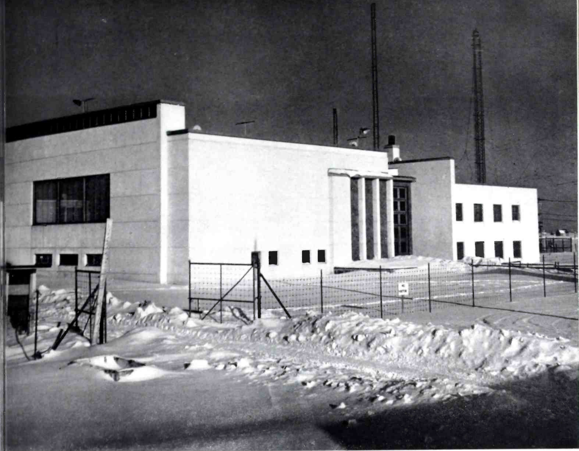
FIG. 2. This modern structure houses three RCA 50 KW transmitters—two Type 50-SW and one Type 50-D.
