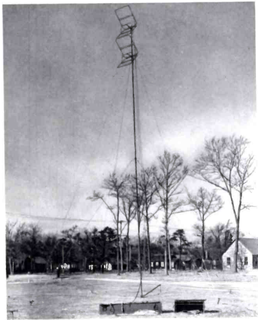
(Above)—Portable antenna system used with the AN/TRC-8 transmitting-receiving equipment designed and built for the Army by RCA.
