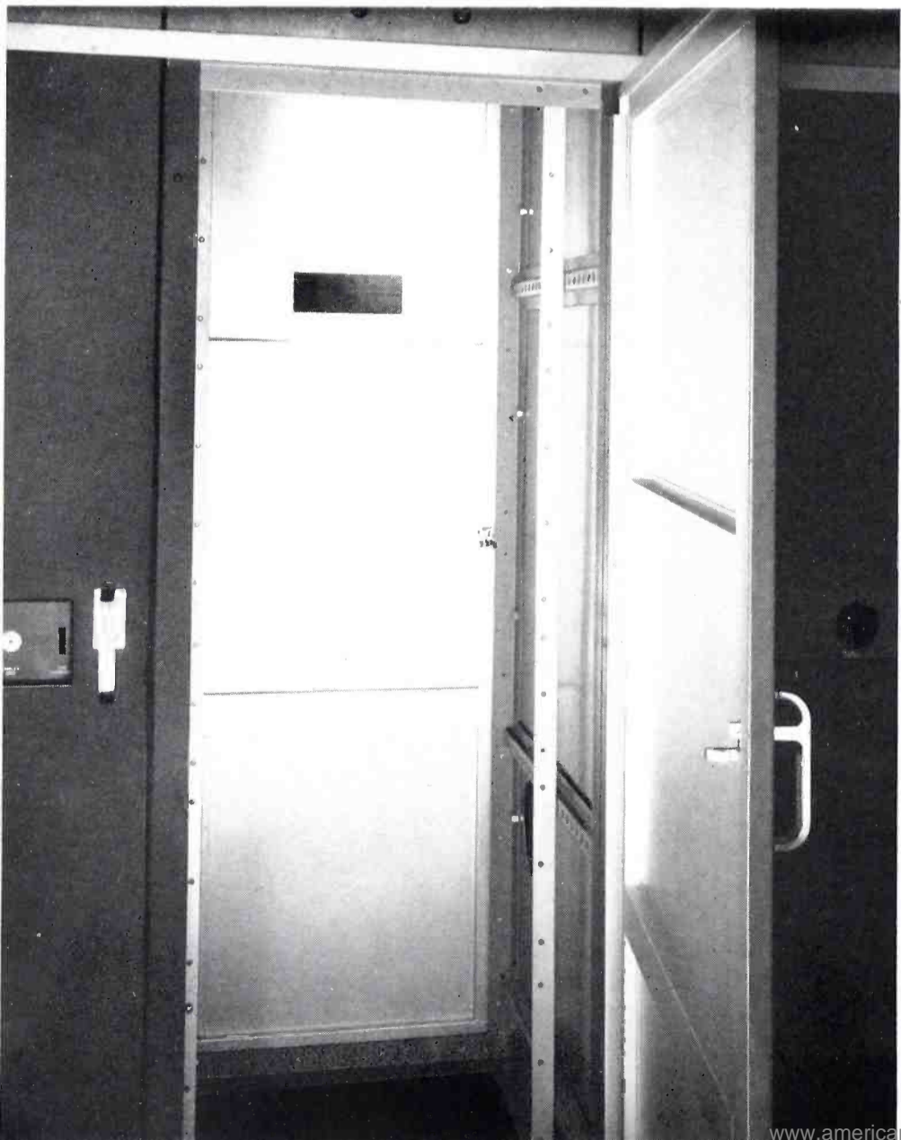
9. INSIDE of one of the cabinet units taken before equipment panels were mounted in place. Vertical arrangement of panels provides good ventilation.
