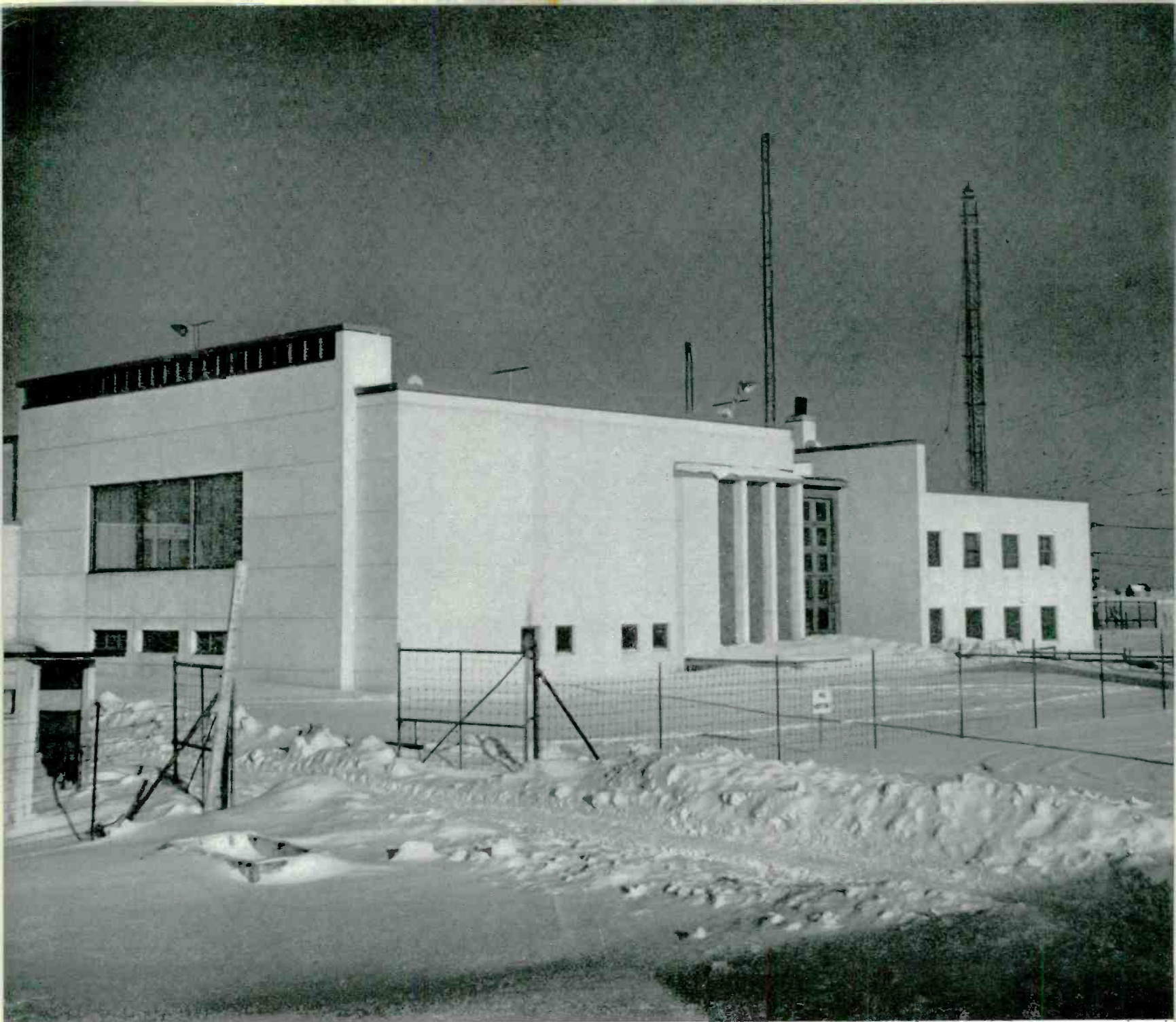
FIG. 2. This modern structure houses three RCA 50 KW transmitters—two Type 50-SW and one Type 50-D.
