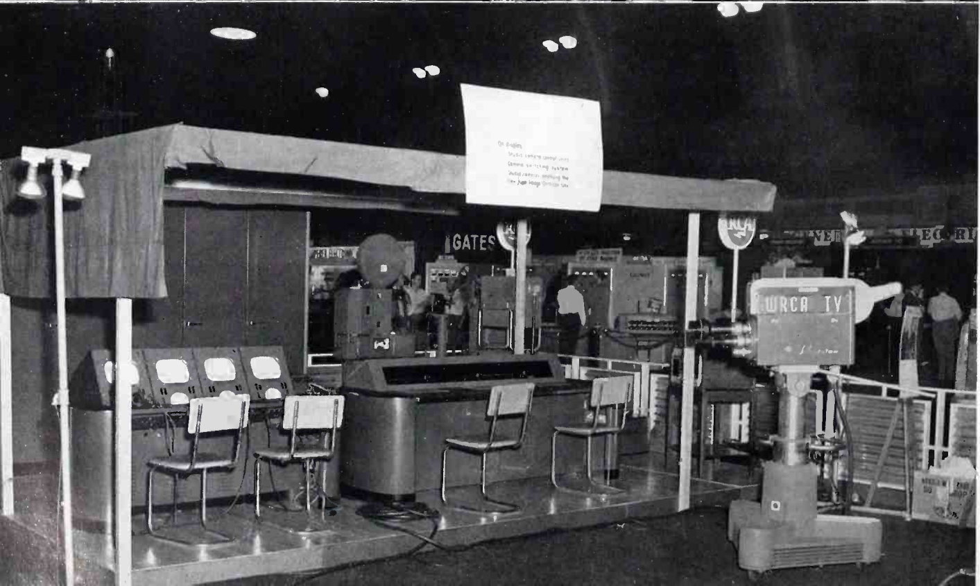
Newest equipment exhibited was this setup of studio-type video units. Under the canopy are new video control and program consoles. In foreground is the new studio camera.
