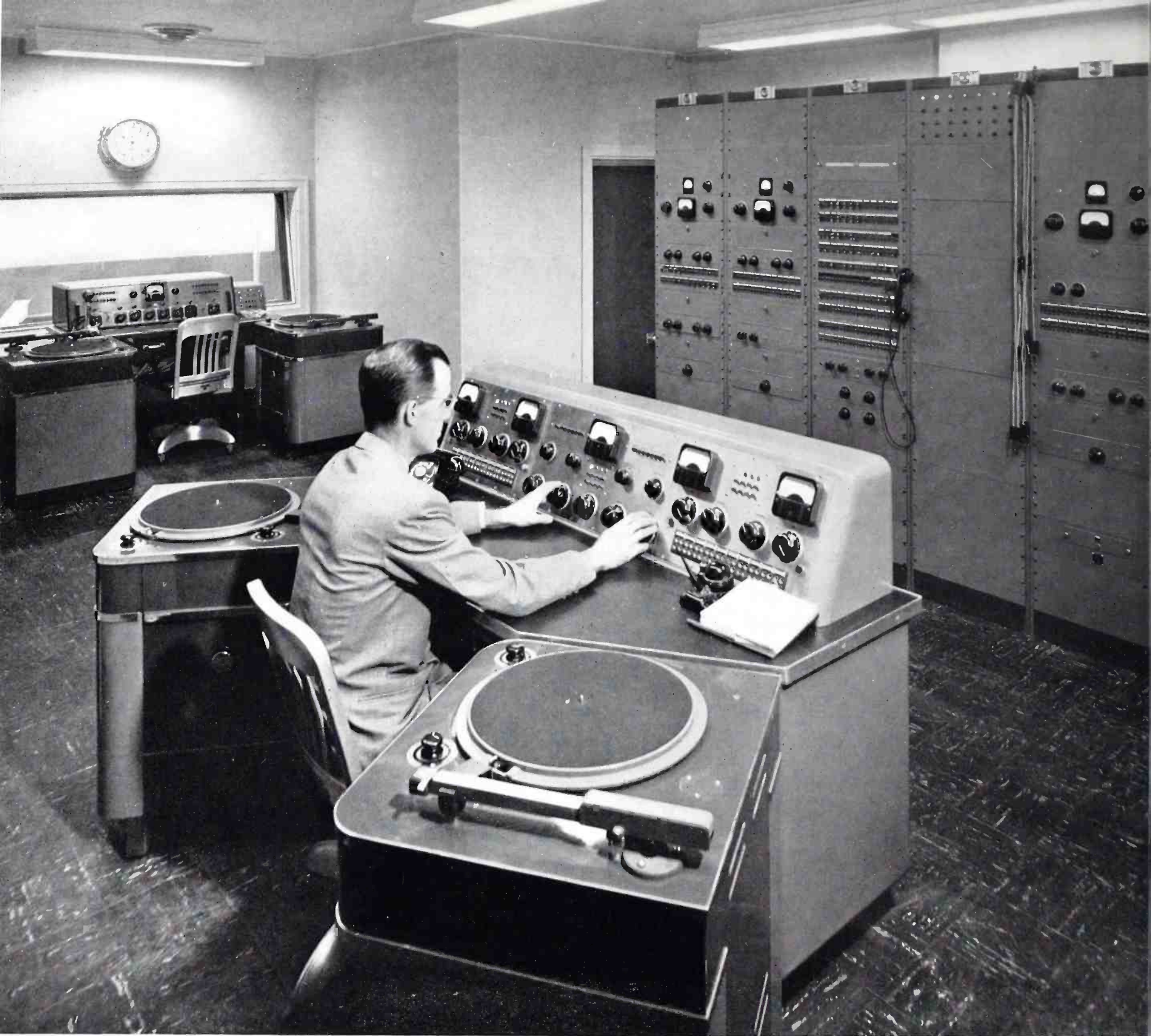
FIG. 1. Master control room of WBAL's new studio installation. R. S. Duncan, Chief Engineer of WBAL, at the control console.
