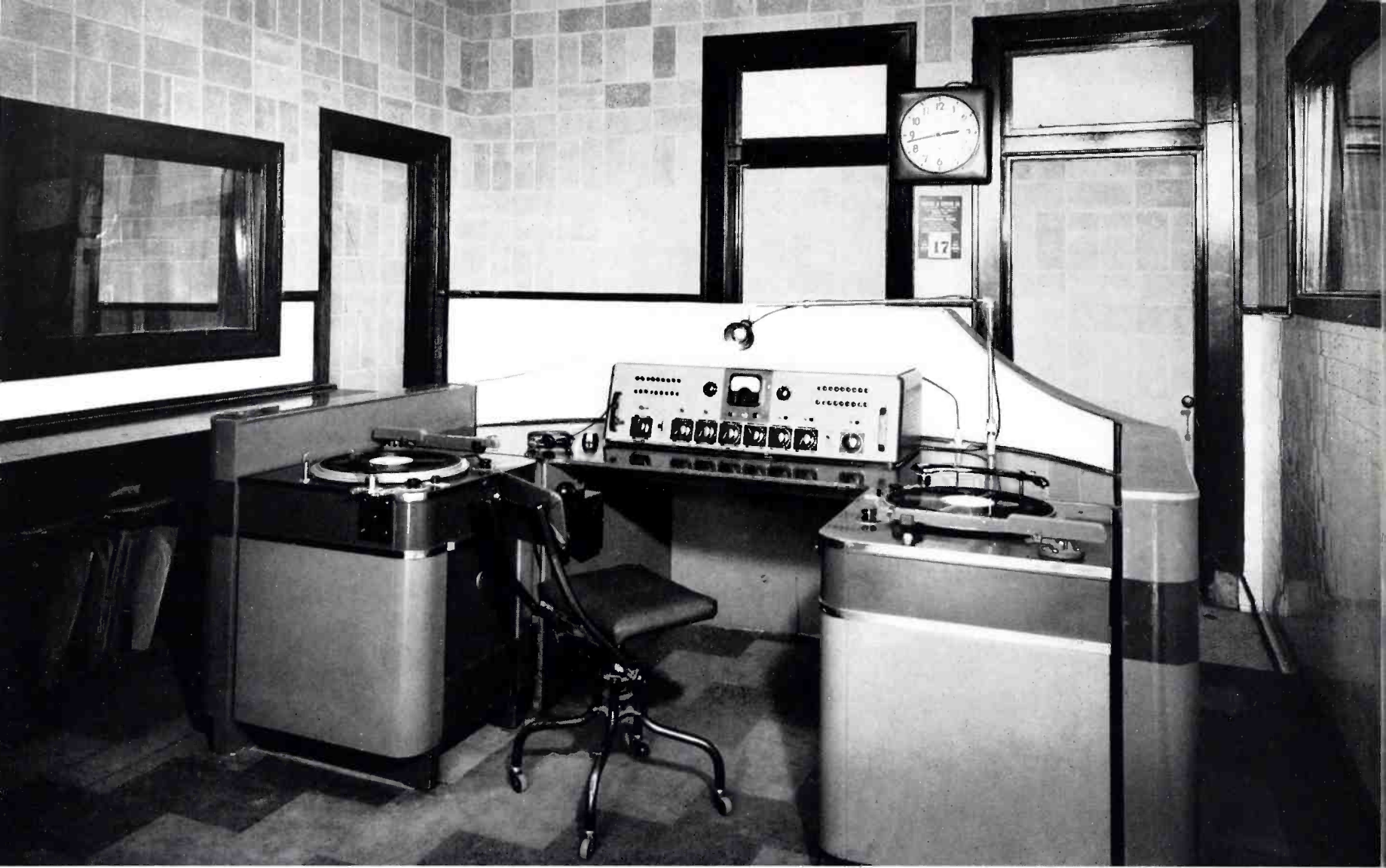
FIG. 1. (Above) Control room of WMOX. The streamlined control console, built by WMOX, has several ingenious features, including a guard wall, which protects the 70-C1 Turntables, an acoustic baffleboard behind the 76-B2 Console, and an 88-A Microphone mounted on a conveniently adjustable pipe-arm.
