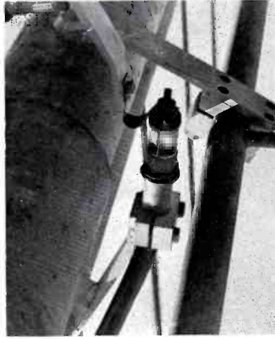
FIG. 14. Feed line clamps and end seal.
