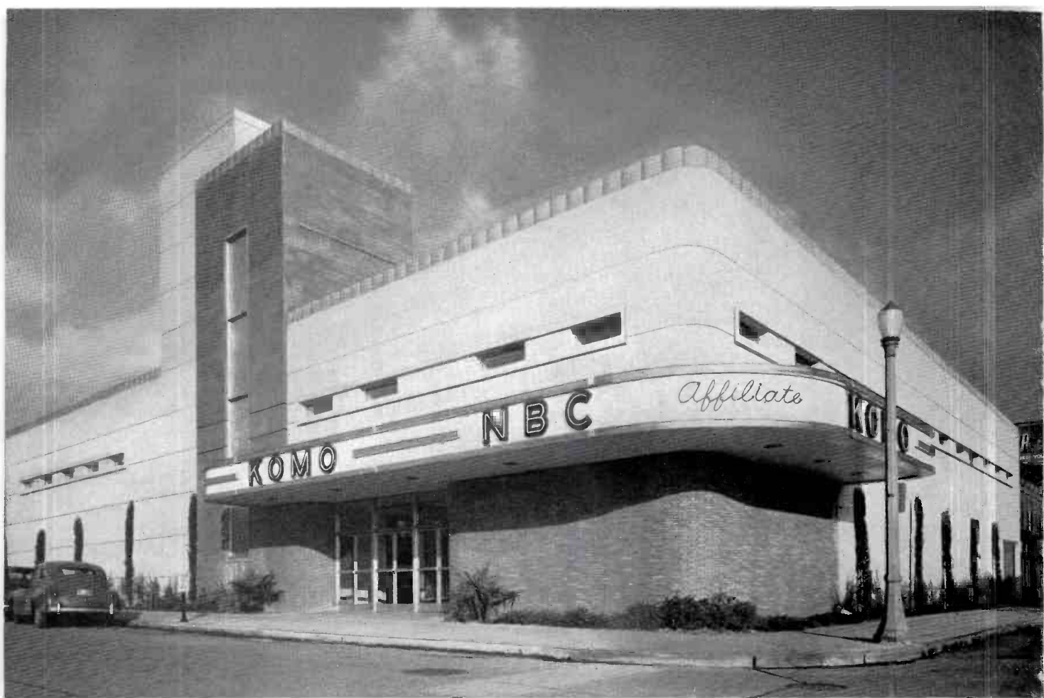
FIG. 3. The complete KOMO studio building is shown above. Of reinforced concrete construction it presently houses six studios, is designed for the addition of another floor if future expansion for FM and TV require it.
