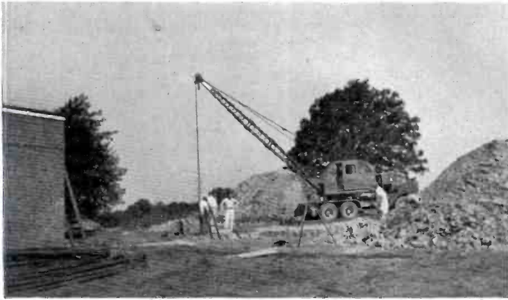
FIG. 4. Excavation for the tower foundation gets under way at WEWS, Cleveland.
