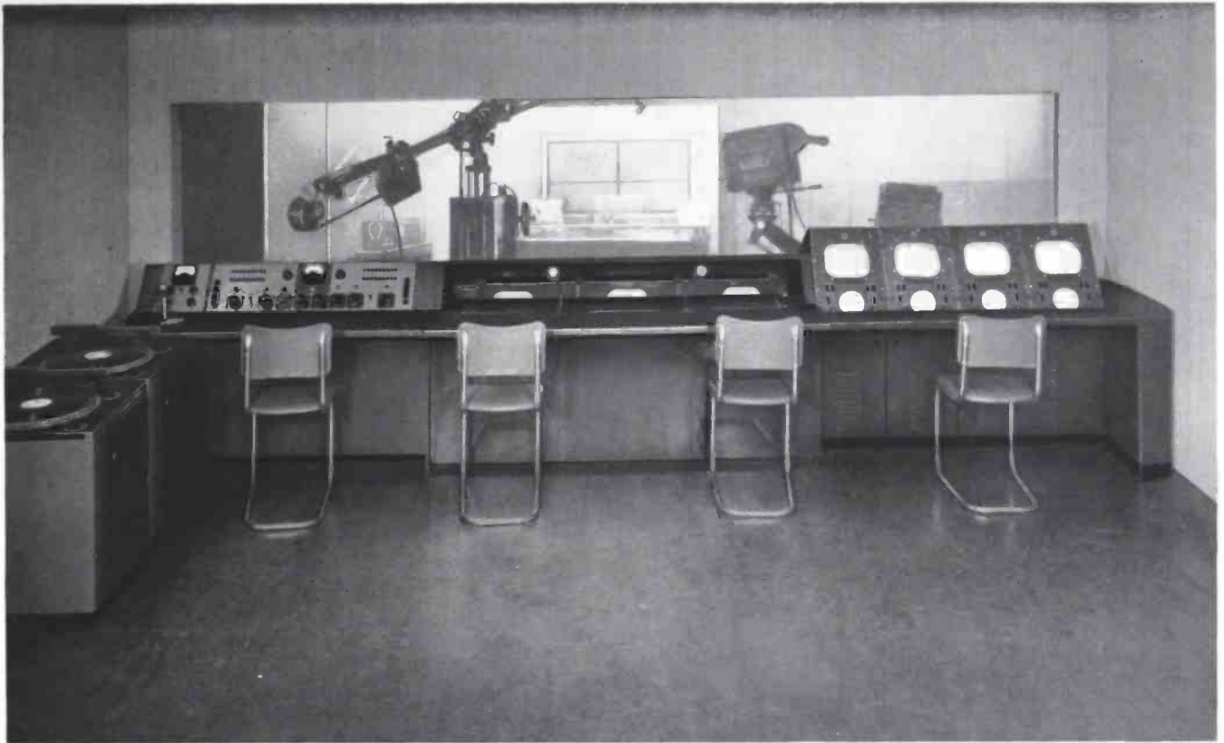
FIG. 29. Studio Control Room of the Type E Layout. This layout employs two control rooms, and features the utilitarian Program Director's Console (center), described in the text. Video Console at right displays pictures from each of three Studio Cameras plus picture on studio output line.
