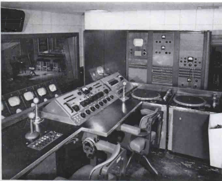
FIG. 22. View of a television studio control room showing video and audio monitoring facilities.
