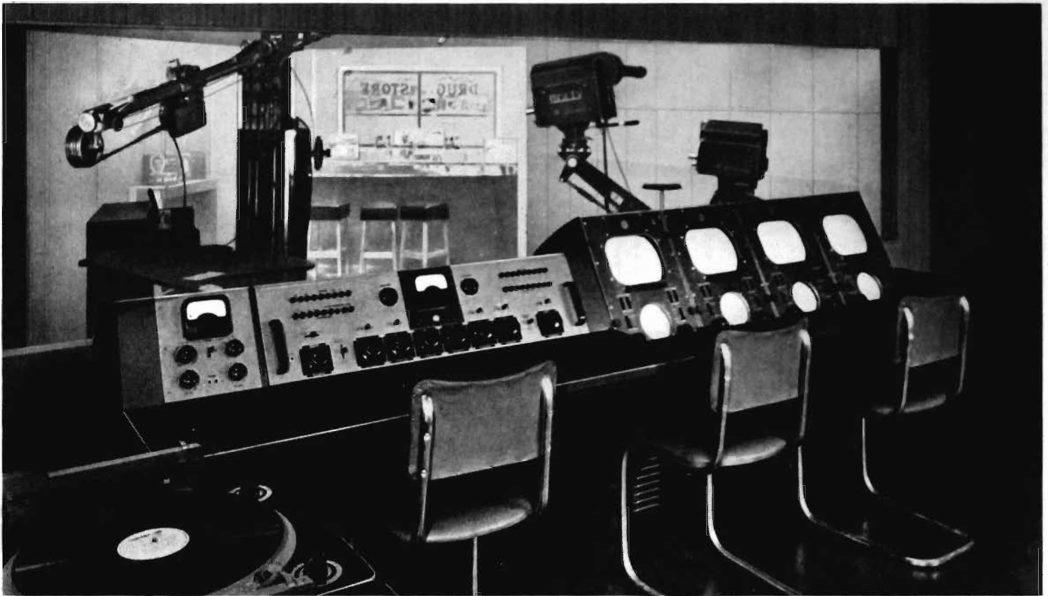
FIG. 25. Studio Control Room of Type D Layout. This layout has a separate control room for the live talent studio, which permits camera rehearsals while remote pickups, network or film shows are being broadcast through master control.
