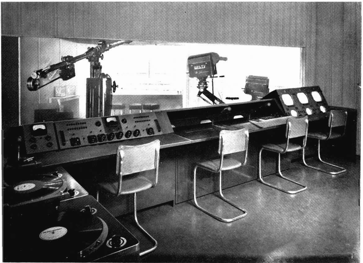
FIG. 32. One of the Studio Control Rooms in the Type F Station. This type station employs two or more studios each with similarly equipped control rooms. Several other physical arrangements of the unit-built control equipment are possible.
