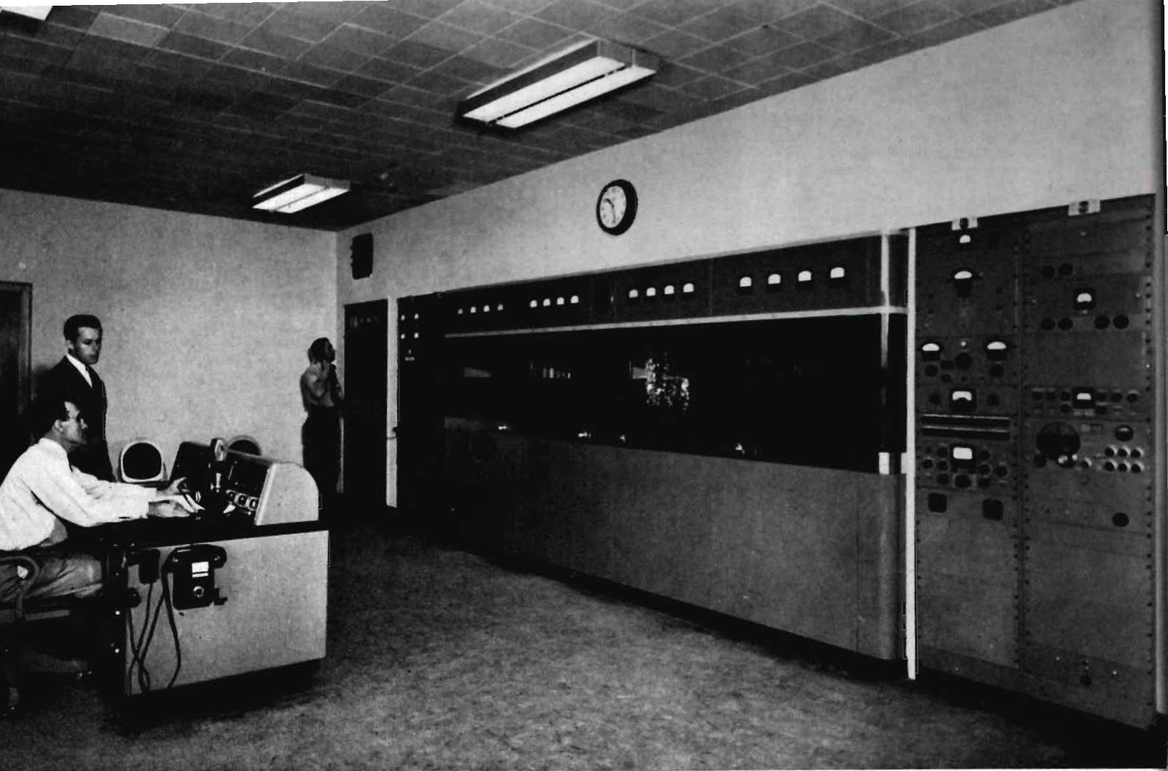
FIG. 3 (above). While Ira A. Smith checks the phasing, W. L. Clements (seated) and W. H. Hamrick watch the RCA BTA-5F transmitter supervisory console. Audio, test, and monitoring equipment are located on the right rack.
